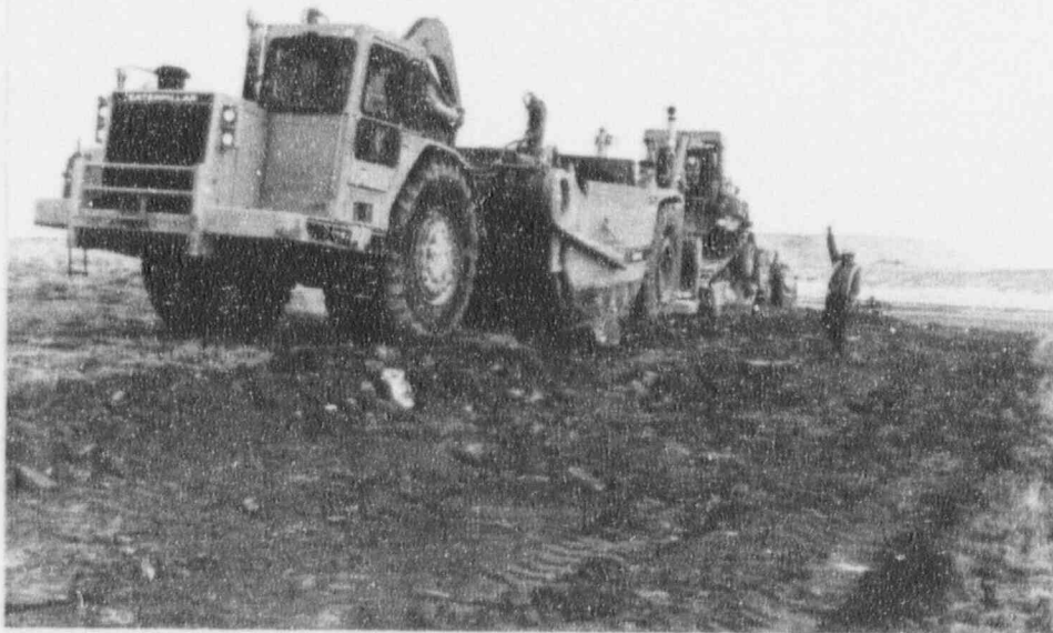
Figure 2-4 Scraper Removing Bladed Windrows
