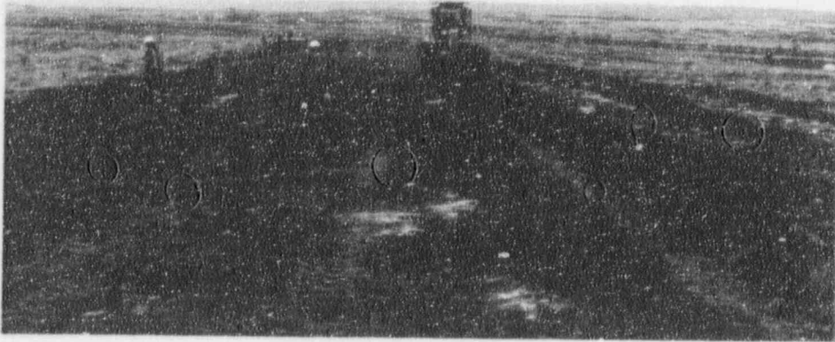
Figure 2-3 Grader Blading Loose Soil in Rock Outcrop Area
