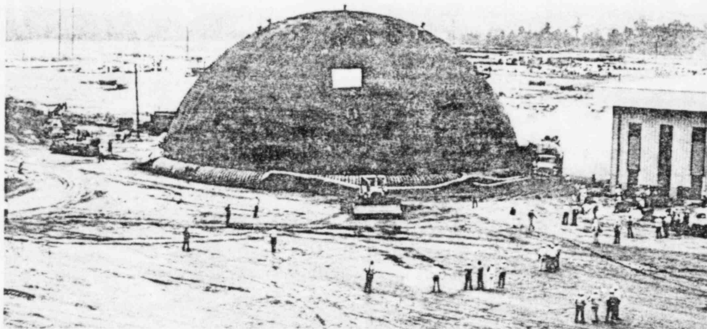
AIR FLOATING CONTAINMENT DOME INTO POSITION
