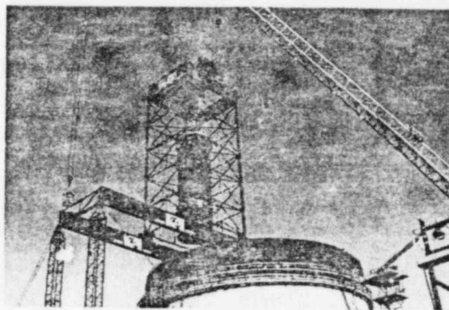
REACTOR VESSEL PLACEMENT
