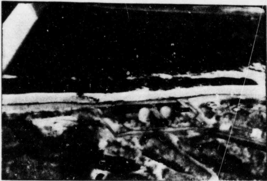
Figure 3. Breached first ridge, second lagoon, and second ridge near the south end of the Cook turbine building. First lagoon is open water. Roll 2, slide #14, 25 February 1982.
