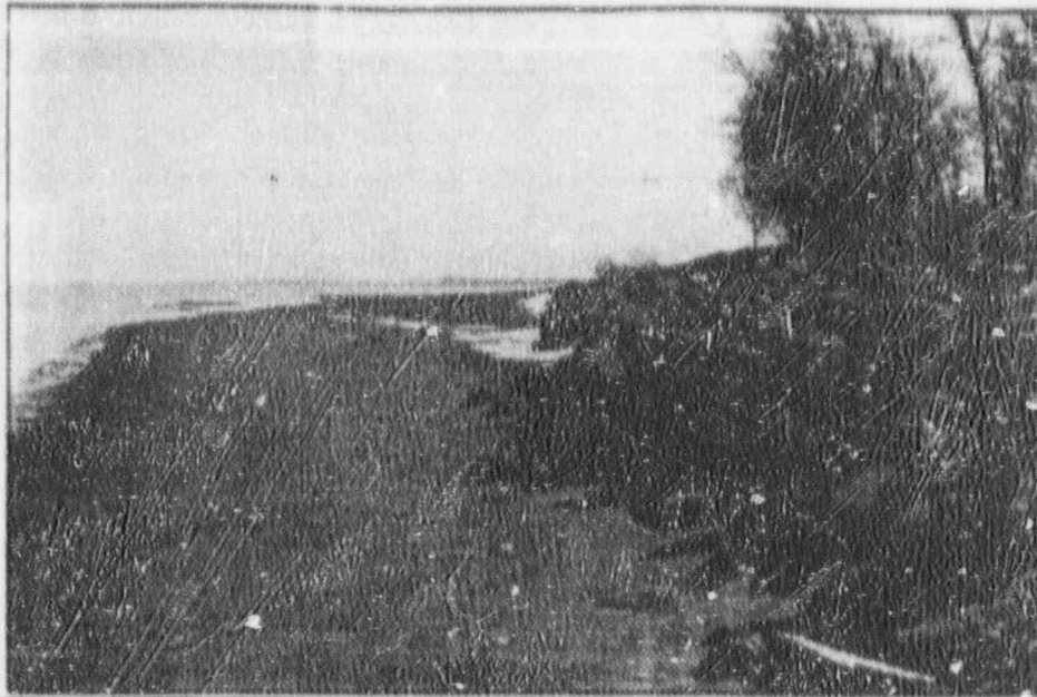
Figure 5-4: The revetment encouraged this beach to form within the first two years. While encouraging beach formation, the revetment also provides a means of flood control and protects the marsh against the wave action of Lake Erie.
