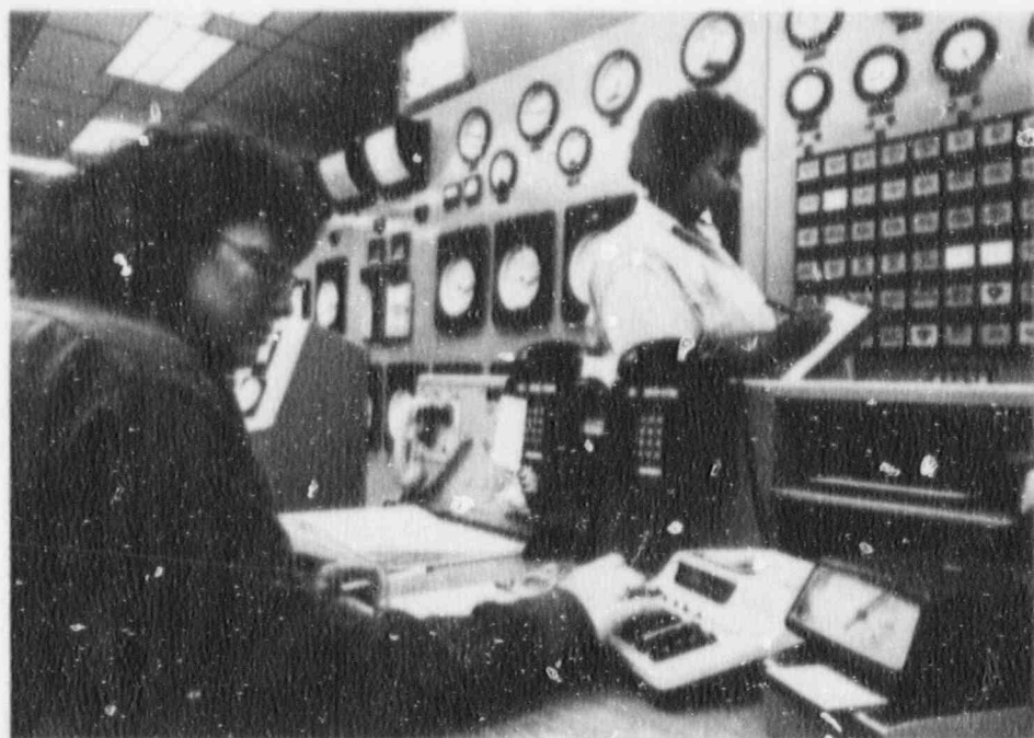
From this North Omaha Station control room, operators oversee the safe and efficient operation of generating units 3 and 4. Together, the five generators at the plant have a combined production capability of 590,100 kilowatts.
