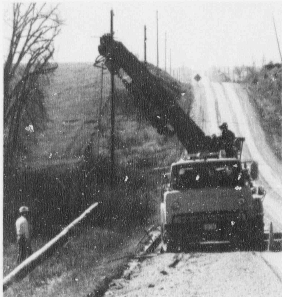
Rebuilding and maintaining the transmission and distribution system throughout the 5,000-square-mile service territory are the responsibilities of OPPD's Electric Operations Division. This crew from Tecumseh replaces an old line on a rural highway in southeastern Nebraska.
