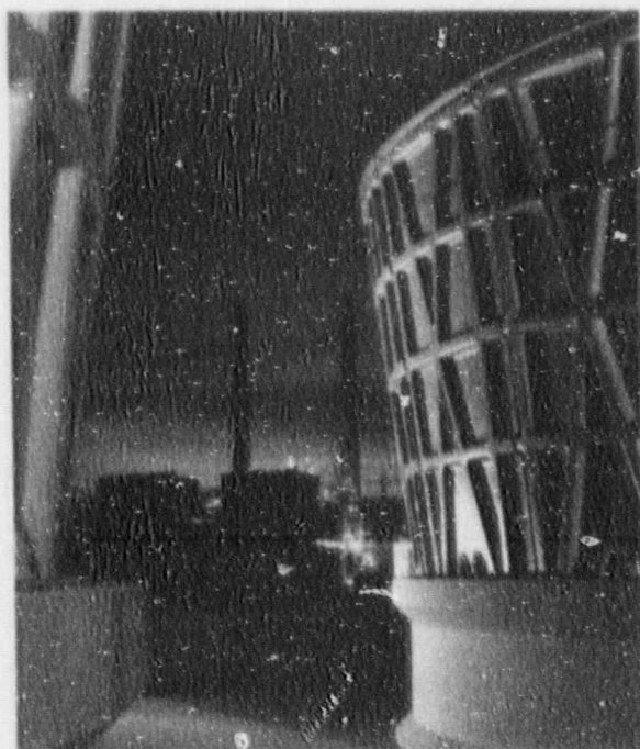
THE STACKS OF BRANDON SHORES ARE SEEN HERE FROM THE DECK OF UNIT 2'S RECENTLY COMPLETED HIGH-EFFICIENCY COOLING TOWER. UNIT 2 IS SCHEDULED TO BE PLACED IN SERVICE IN THE SPRING OF 1991.
