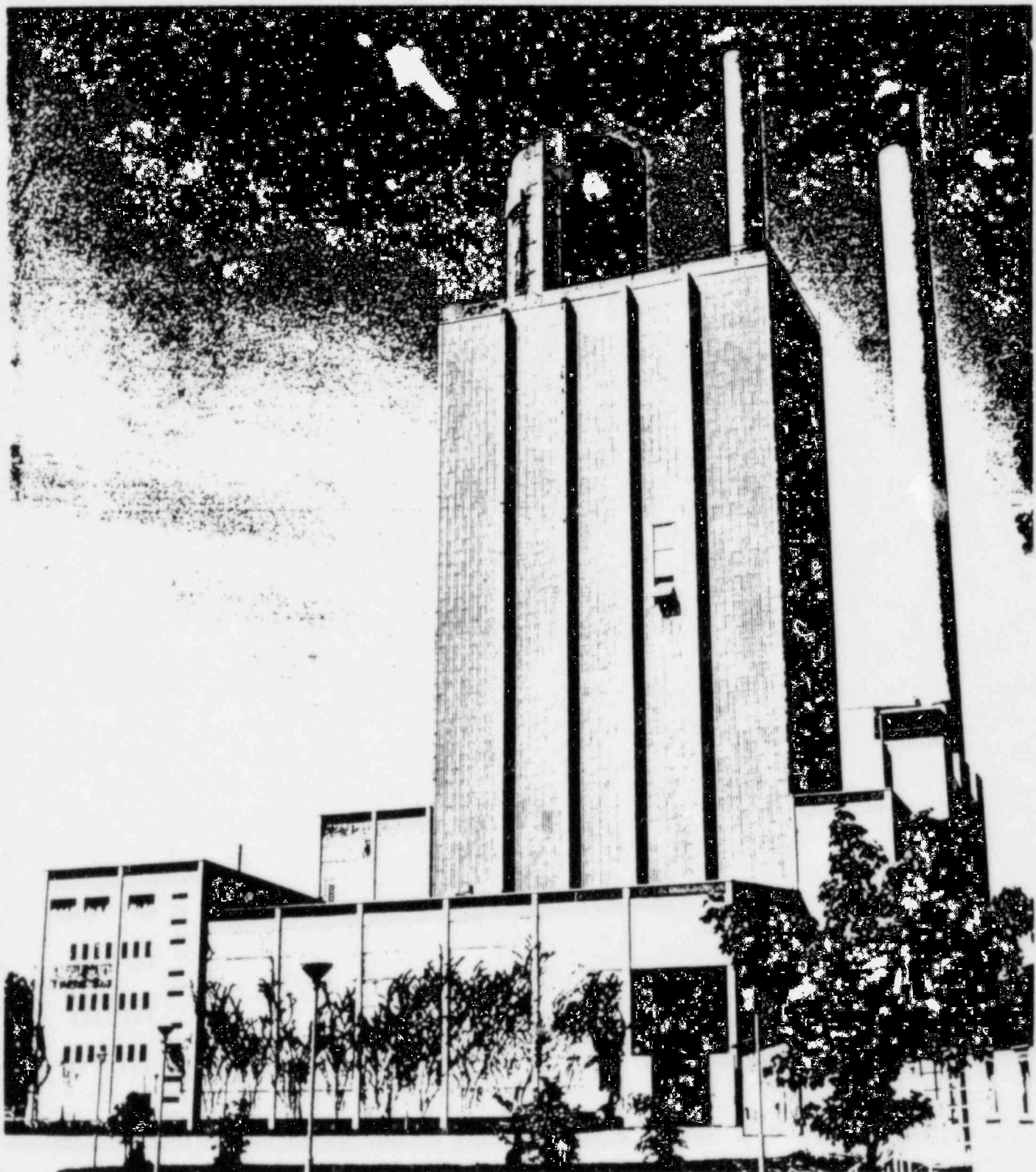
Figure 10 General View of the Marviken Test Facility
