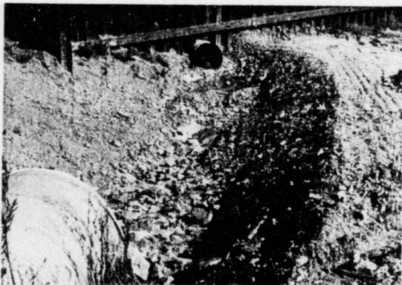
Figure A-29. Downstream sedimentation study site at Station 8, 13 August 1980. This is the final configuration of the altered stream bed. No sediment accumulation was noticeable on the riprapped stream bed.
