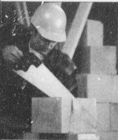
In 1993, our Company hosted a demonstration project for autoclaved cellular concrete – a lightweight building material made primarily from power plant fly ash.
