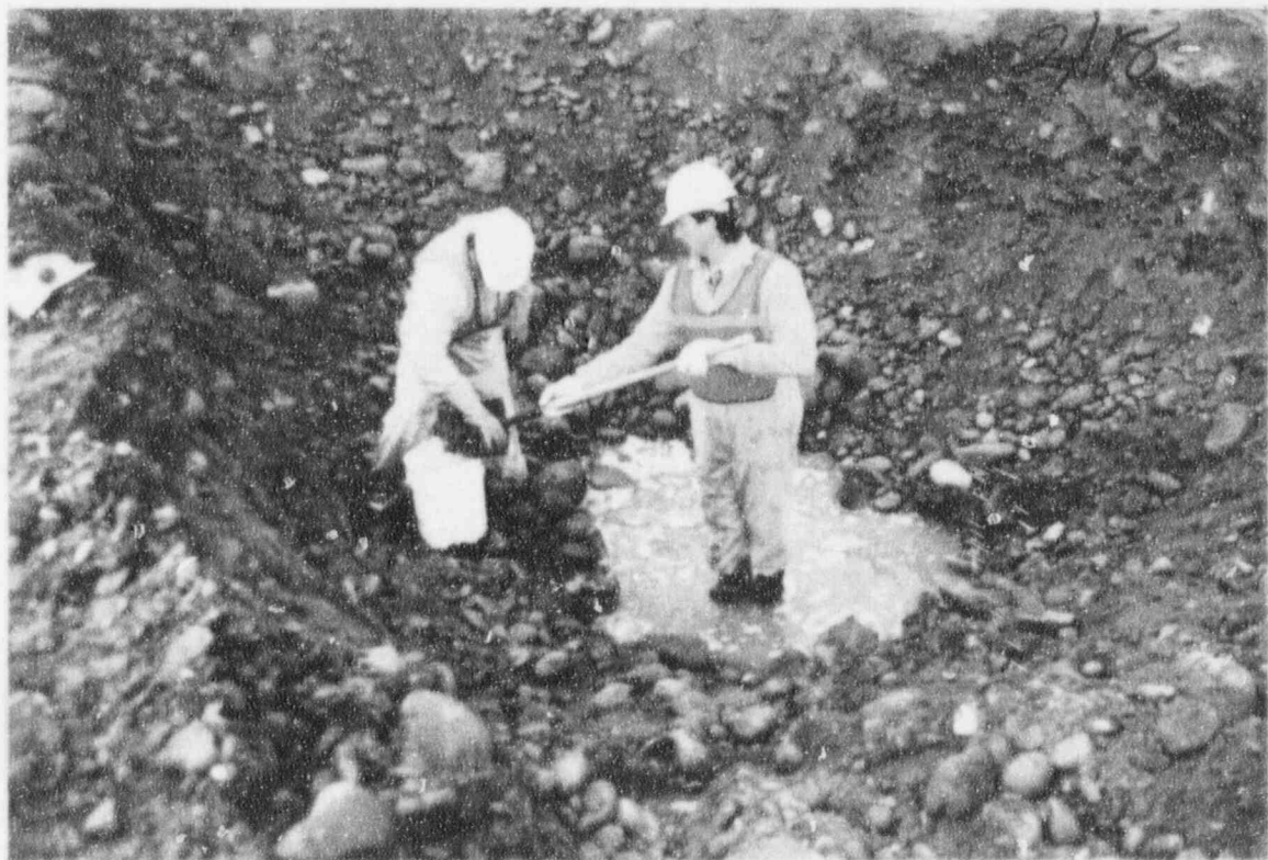
TP M-CF-20. Bottom of test pit in sand, gravel and cobbles. Ground water encountered at a shallow depth.
