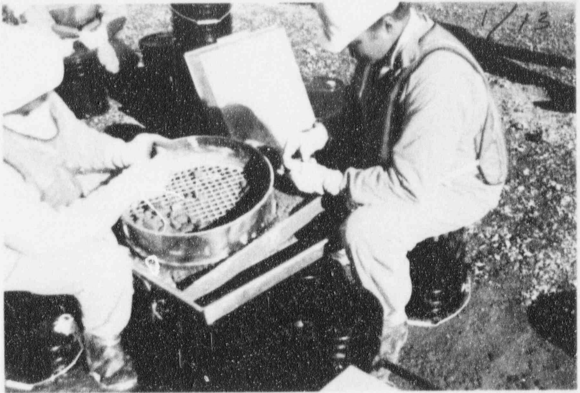
Screening semi-dry samples.
