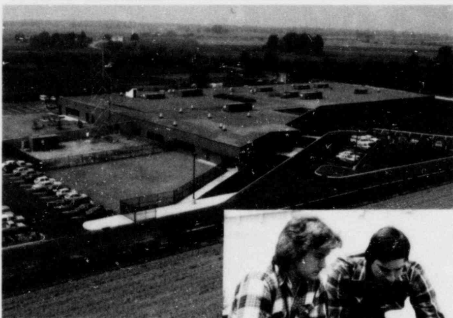
A broad curriculum that covers the various aspects of nuclear operations is provided at the Nuclear Training Center. Dedication of the Center is planned to take place in April 1983.
