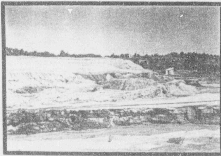
Figure 1-13. Eroded Slopes of the Vanadium Pile. Note cutbank of Montezuma Creek in foreground. Photo dated 11 September 1961.
