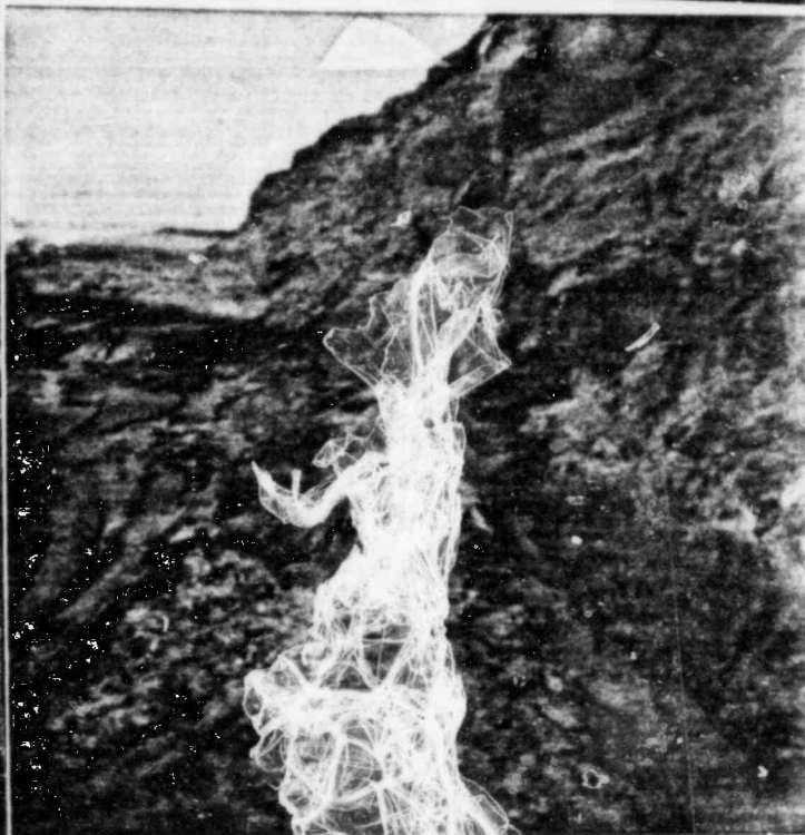
11-11-80 after Slush Grout Sta 4+00-4+50
