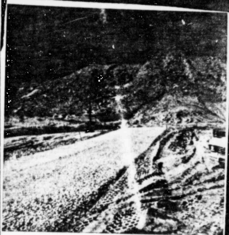
Blanket Draw Compacted 10-7-80
