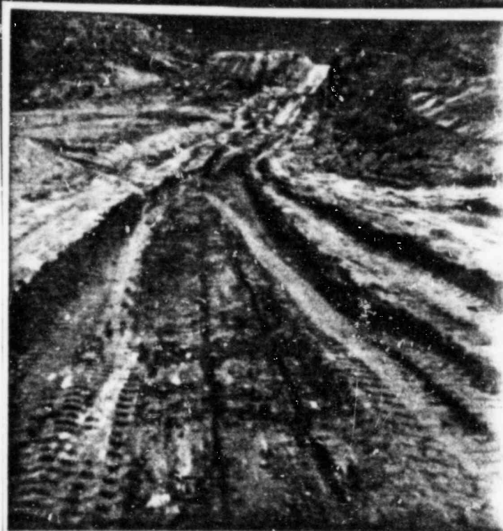
KEYWAY TRENCH LOOKING EAST
