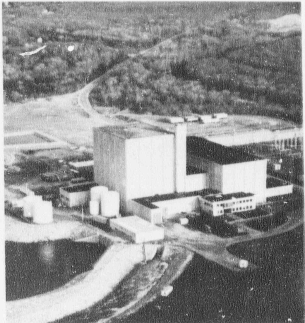
OIG inspectors addressed emergency planning concerns at the Pilgrim Nuclear Power Station.
