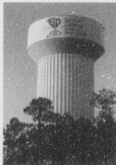
This one-million gallon elevated water storage tank, located between Moncks Corner and Summerville, is part of the Santee Cooper Regional Water System.
