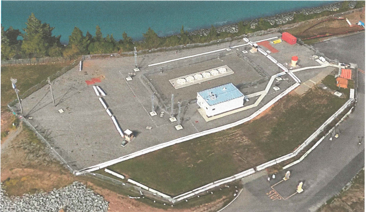
Figure 1 - Aerial view of HB ISFSI
