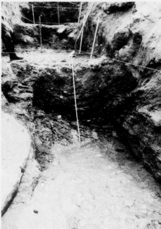
PHOTOS OF SLUMPED SOIL OVER FAULT 2817-2819 ON SOUTH EMBANKMENT. NOTE CONTINUITY OF IRON-STAINED LAYERS OF SOIL
