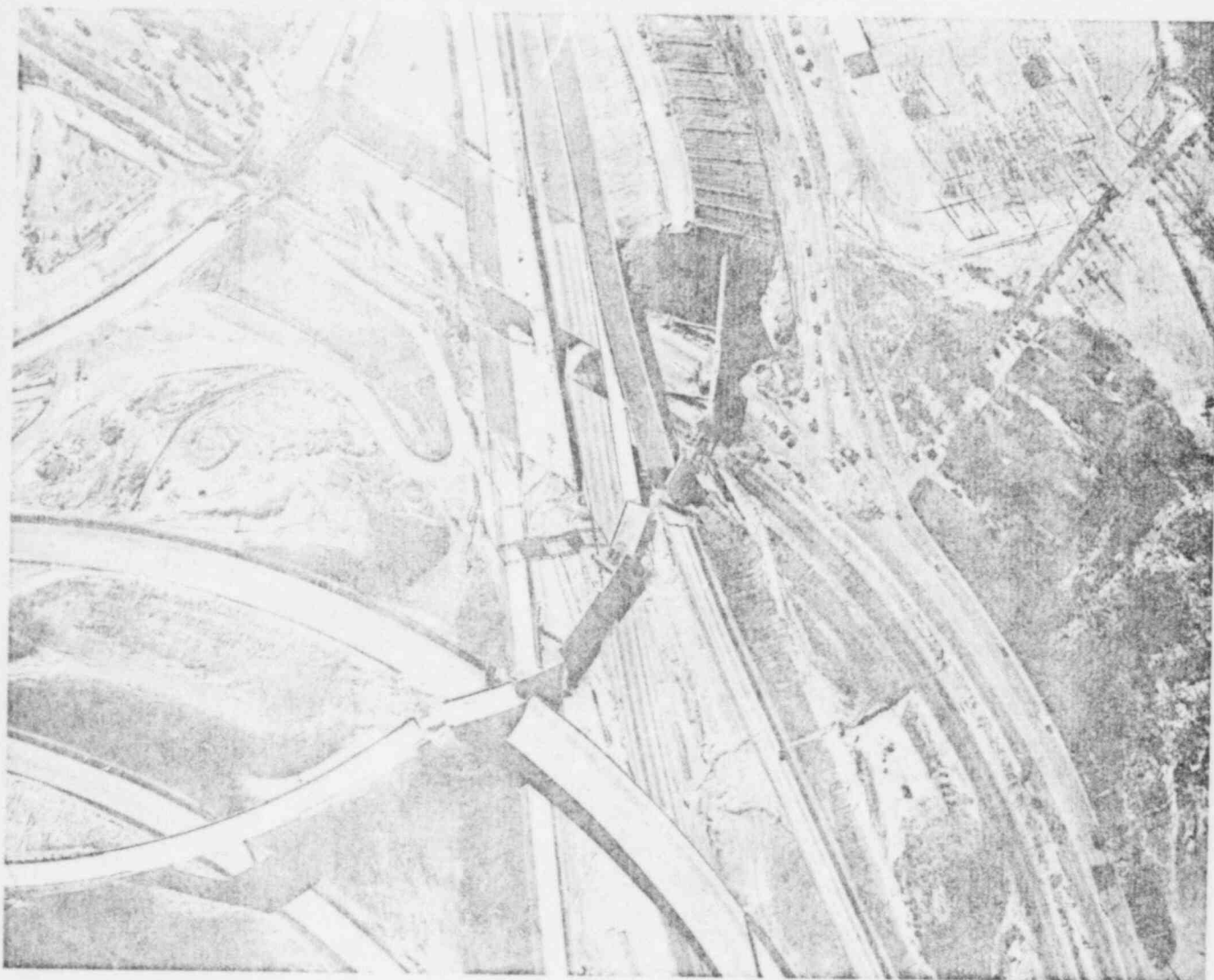
HIGHWAY 5 INTERCHANGE FOLLOWING THE SAN FERNANDO EARTHQUAKE OF FEBRUARY 9, 1971--AN AERIAL VIEW (Recommendation No. 2)
