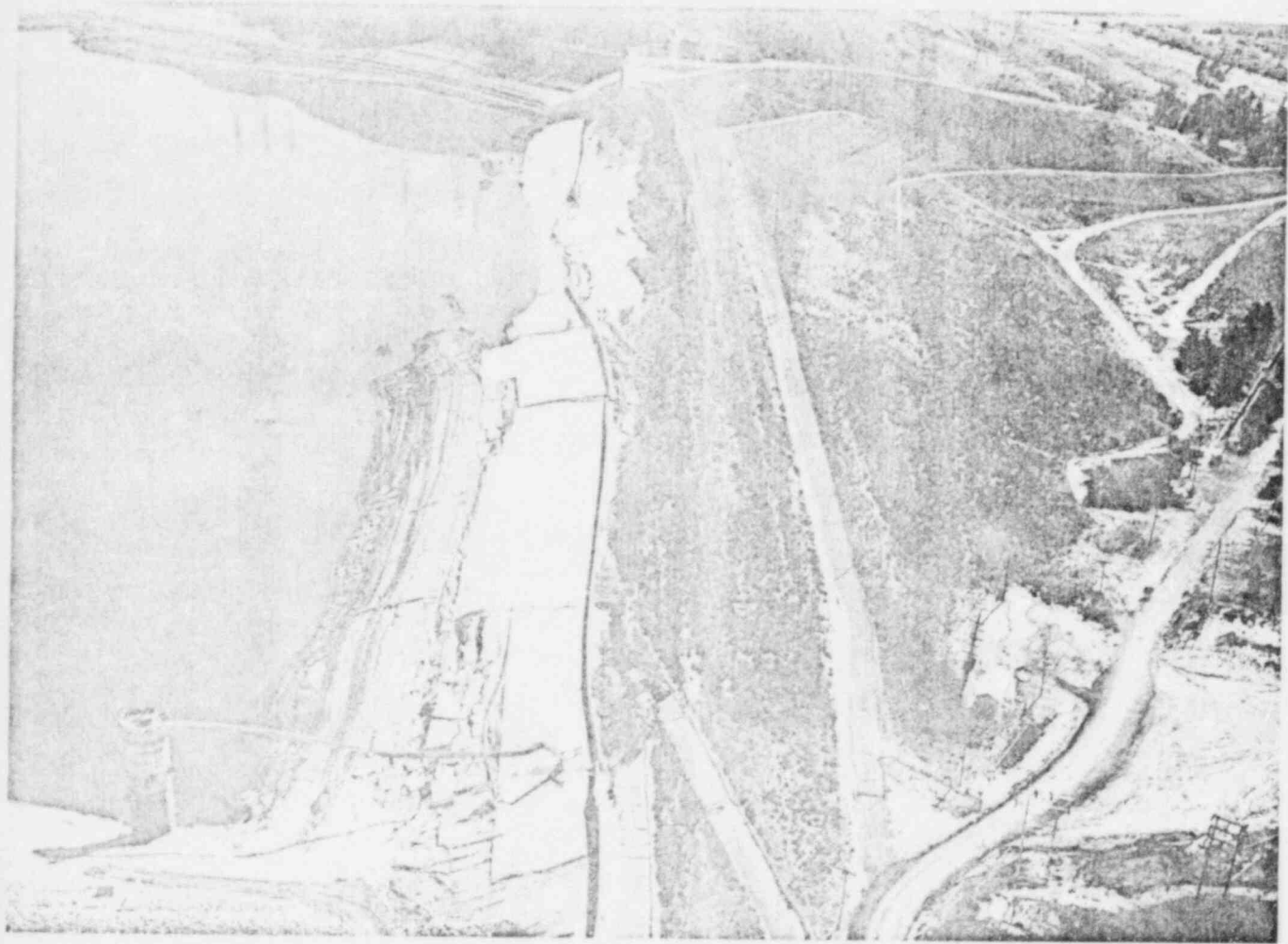
LOWER SAN FERNANDO DAM, LOS ANGELES COUNTY (Recommendation No. 4)
