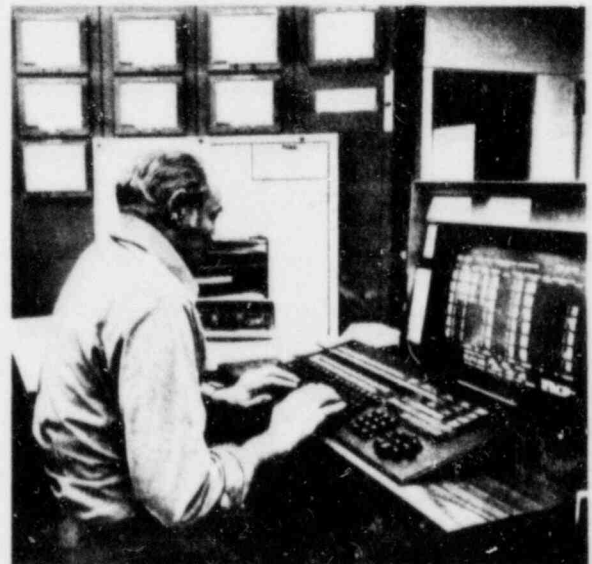
In the Energy Control Center, computers monitor power plant operations, are used for remote control of substation switching and eventually will control generating units.
