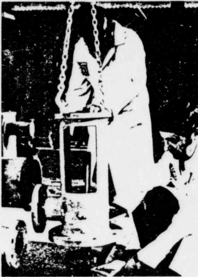
Figure 8-1. INSTALLING THE DISCHARGE HEAD
