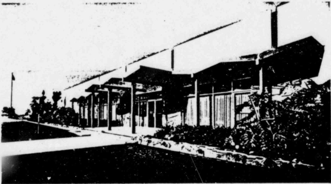
Vertical Pump Division Offices and Plant, City of Industry, California
