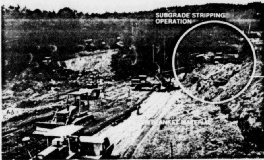
PHOTO 3 OVERLAY CONSTRUCTION AT EL. 1240 (9-4-81)
