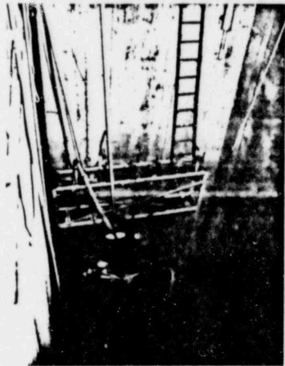
FIG. 30 SECOND-STAGE LIFT FOR REMOVAL OF RUST AND WATER FROM CUTUP POOL
