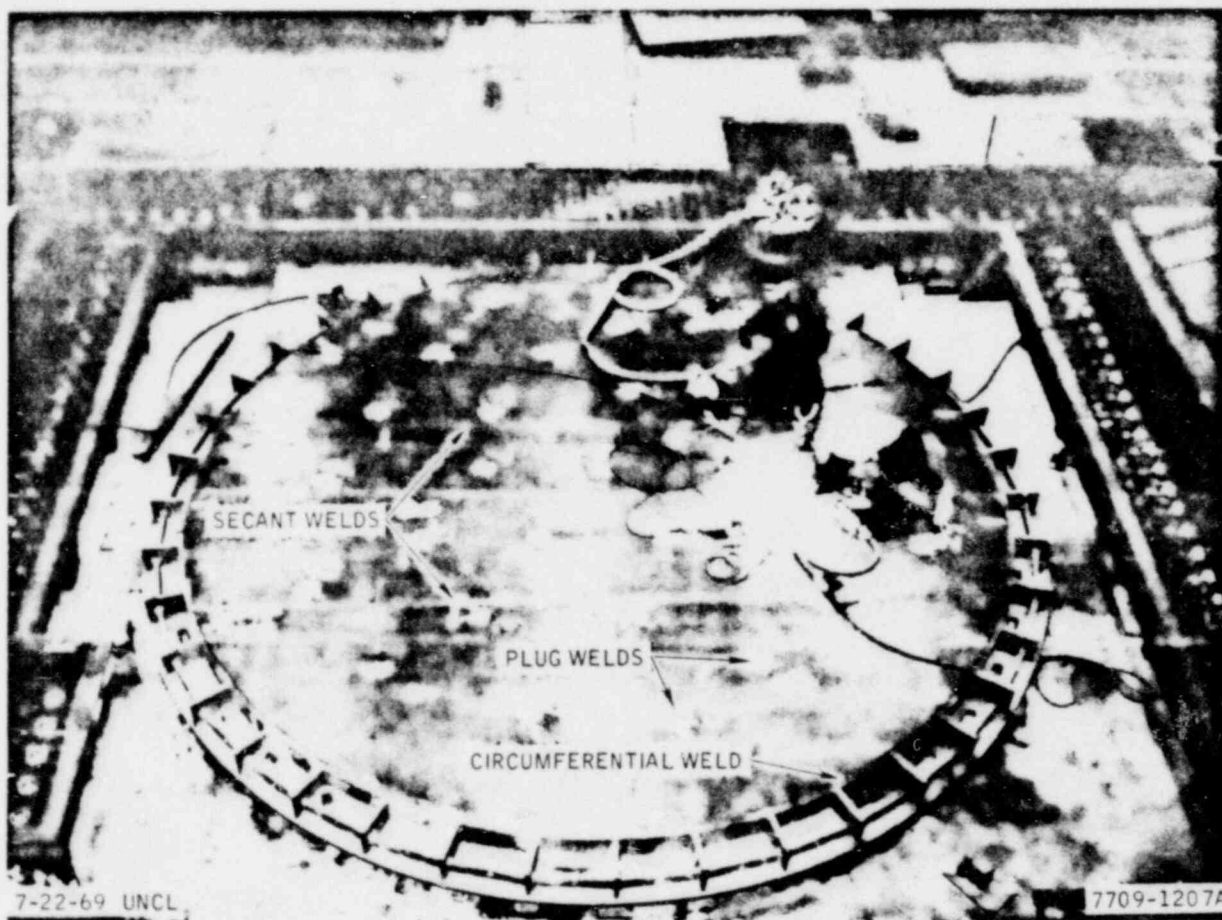
Figure 6-20. Welding of Cover-Plate
