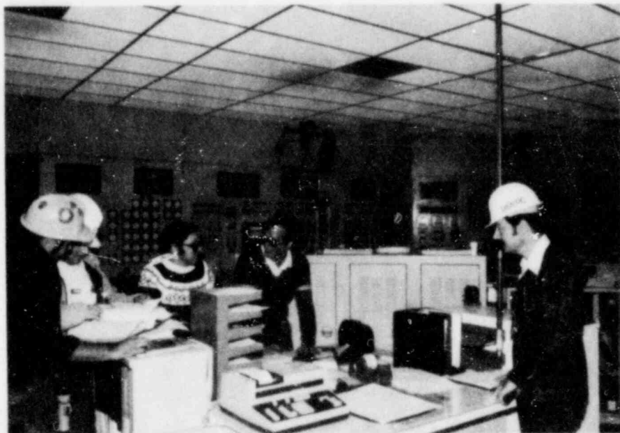
At right is Tom Tongue, senior resident inspector at the Dresden (Ill.) nuclear power plant, looking in on the control room during inspection tour of the plant.
