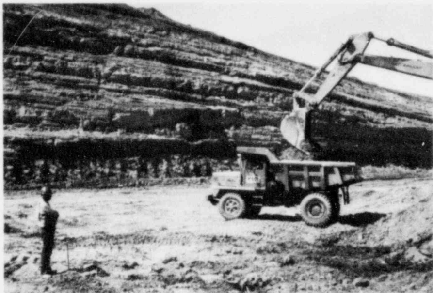
The worker at left is using instruments to probe for radioactivity during open pit mining for uranium. Sandstone deposits break up into sand during the mining process and small amounts of radon-222 escape into the atmosphere. NRC sponsors research to measure the quantity of radon released from these kinds of operations.
