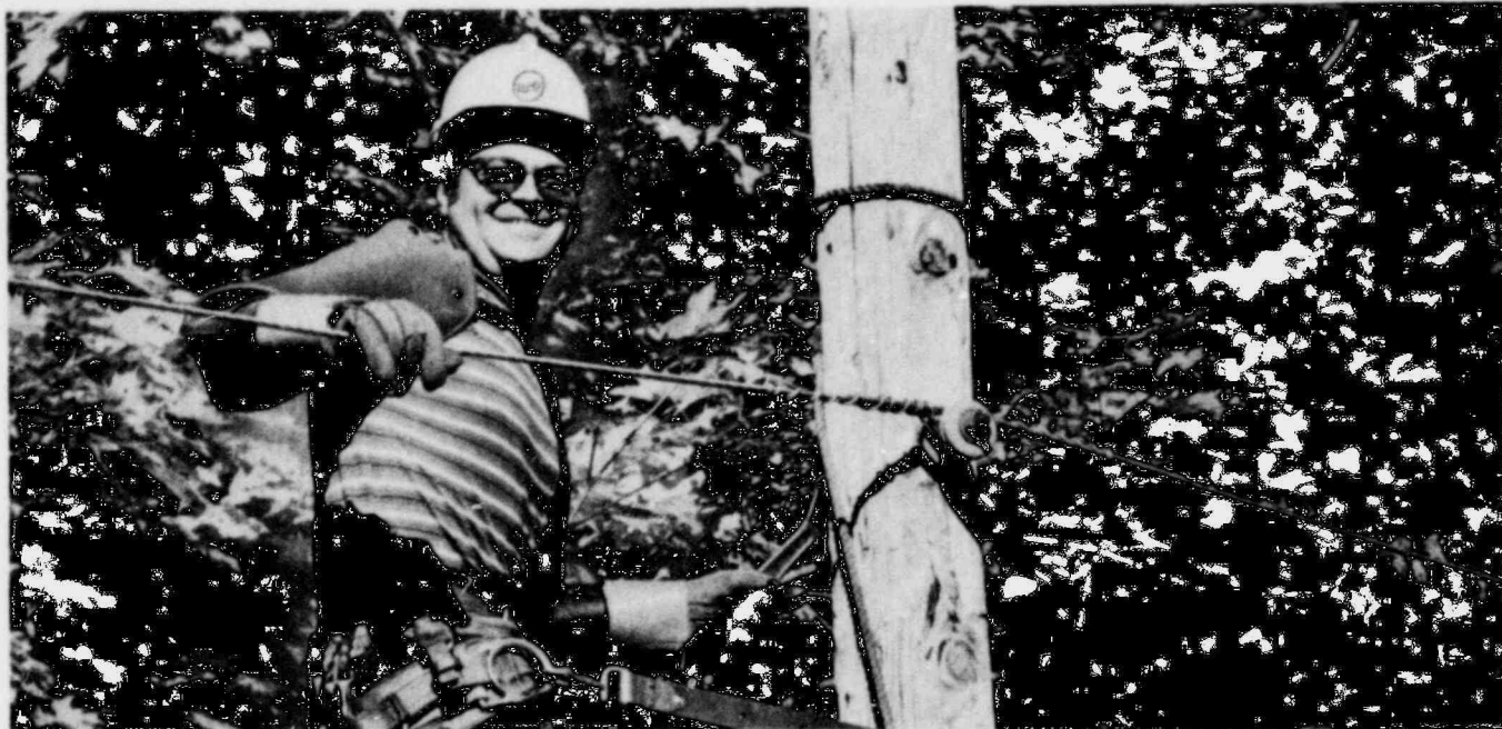
Line mechanic Gerald Liebetau (top photo) helps maintain electric service in the West Bend area. Computer operator Faye Mirr (bottom photo) supplies and stores countless bits of company information.
