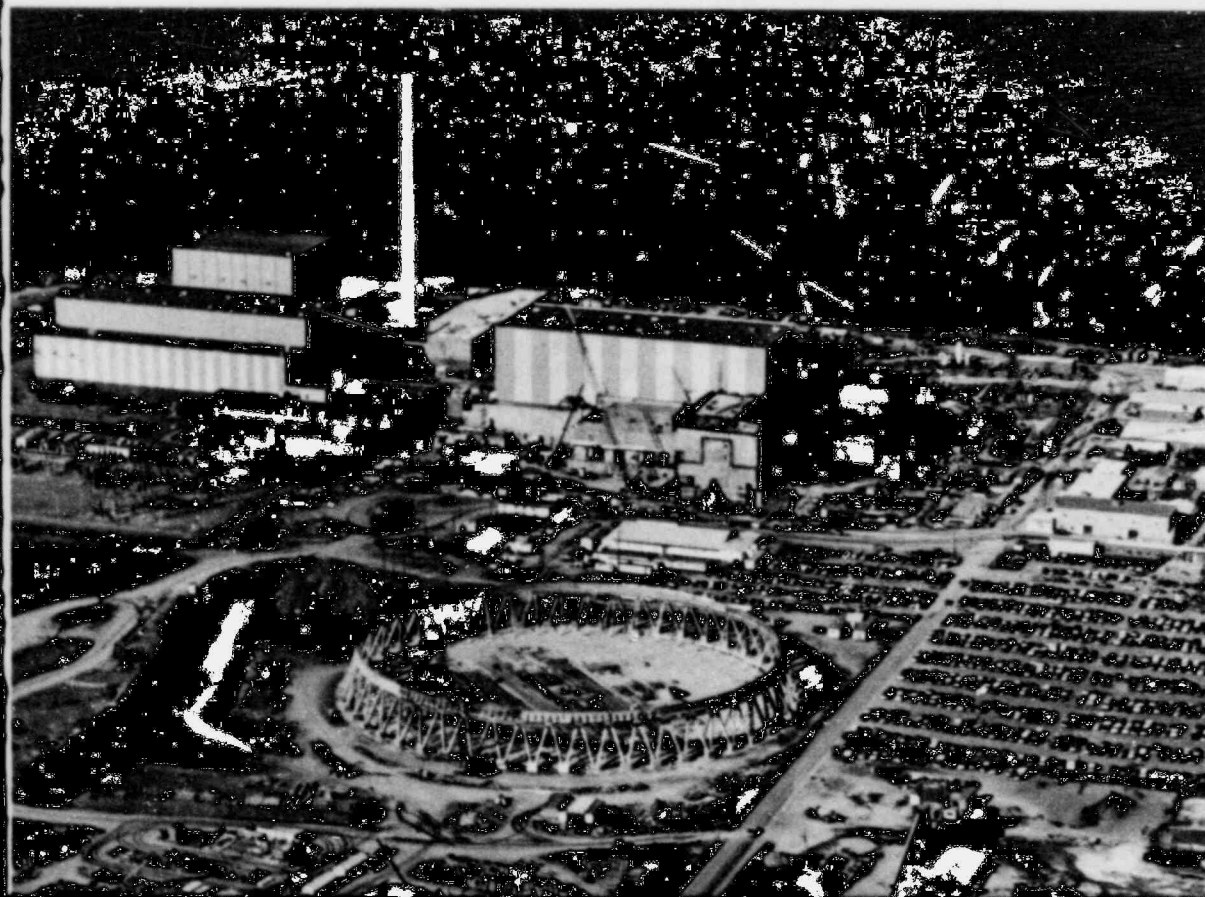
Nine Mile Point Nuclear Unit No. 2, center, is alive with construction activity in this aerial view of Lake Ontario shoreline east of Oswego. Cranes hover over reactor containment structure, at right of station, while huge circular base to support cooling tower is visible in foreground. Building and stack at left are for Unit No. 1, in service since 1969.
