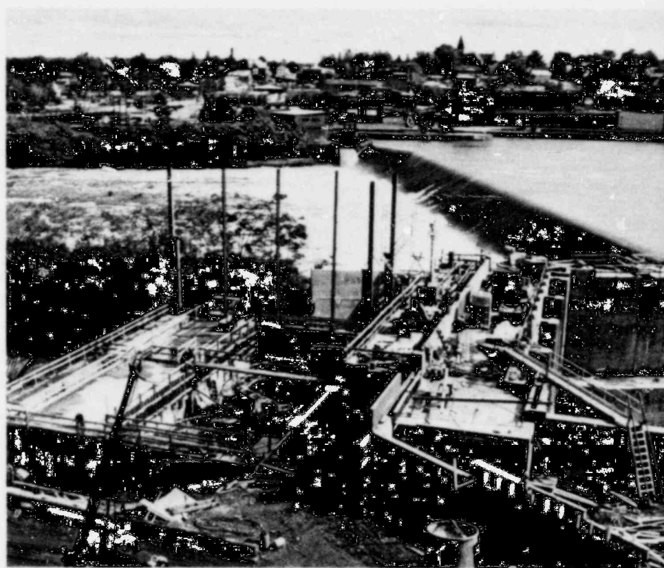
View of Granby Hydro Station under construction on Oswego River shows just-completed powerhouse substructure, left, and intake and forebay complex at right. Targeted for early 1983 startup at 10,000 kilowatts, Granby is among first of projects taking shape in Niagara Mohawk's extensive hydro expansion and development into the 1990s on upper New York State waterways.
