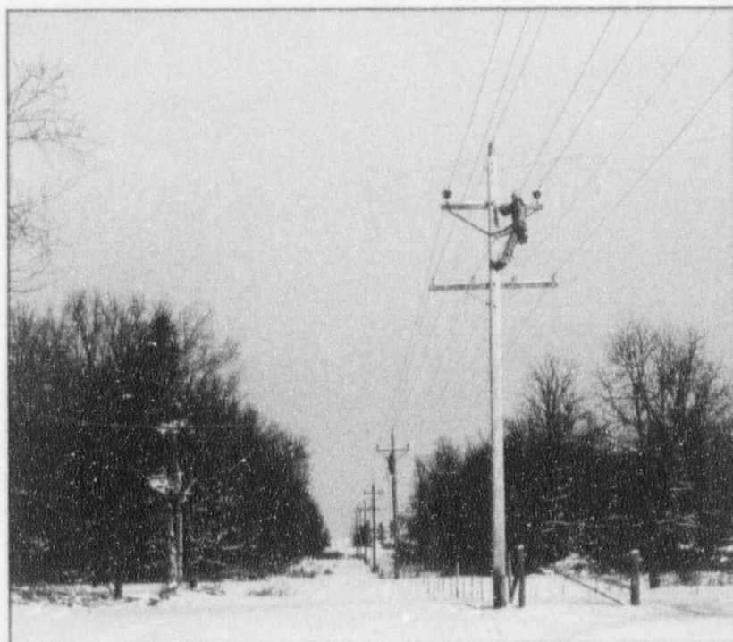
Maquoketa Valley REC crews tighten hardware on CIPCO's Backbone 34.5 kV Tap. ▼
