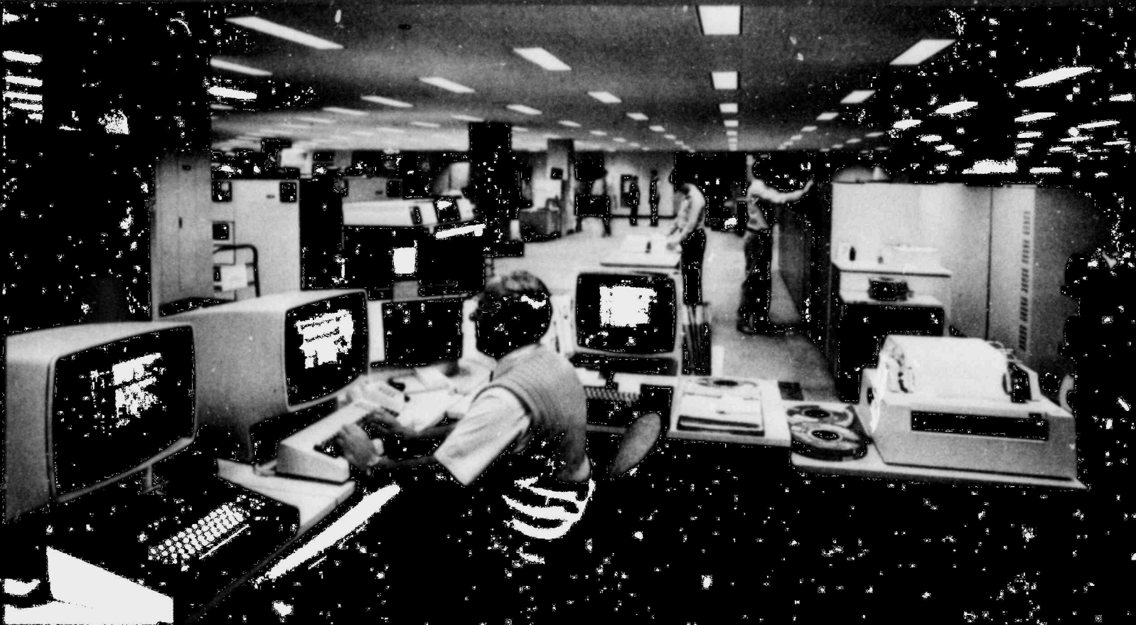
This computer room on Level 21 of the new corporate headquarters building in Newark is the heart and nerve center of the Company's growing computer capability. The room houses the large main computer and associated equipment, employed in the new customer information system as well as in other programs, systems and projects and the development of computer applications.
