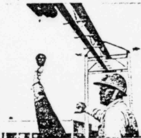
Husky electric crane handles poles with greatest of ease at Miami's new Northeast Yard.
