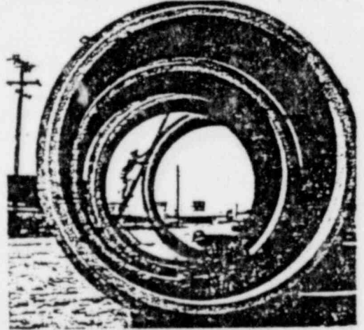
New Port Everglades' circulating water pipe can handle twice the output of Miami's water system.
