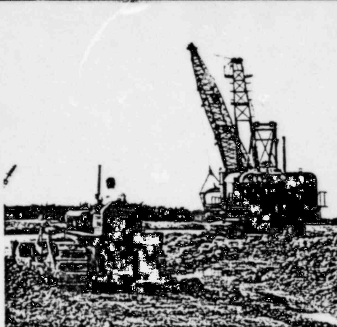
Atomic power units are being considered for installation at Turkey Point, a new plant site being carved from swampland in South Dade County.
