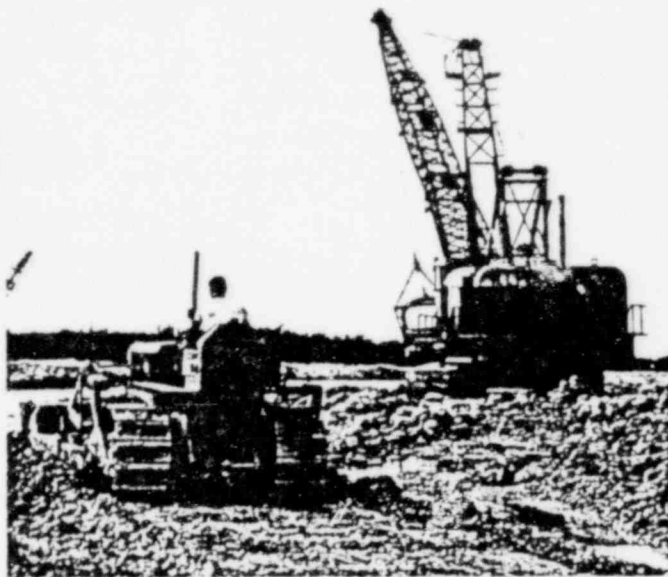
Atomic power units are being considered for installation at Turkey Point, a new plant site being carved from swampland in South Dade County.
