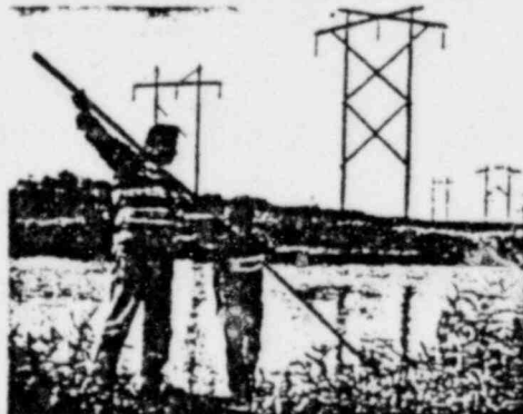
New cross-state line spans the Everglades and here parallels an older, less powerful one.
