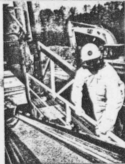
Technician Otis Malcom, Jr., monitors the operation of a mobile stabilization and fixation unit at a site in North Carolina. Westinghouse Remediation Services uses the unit to process chemical waste with cement, transforming it into a non-hazardous composite.
