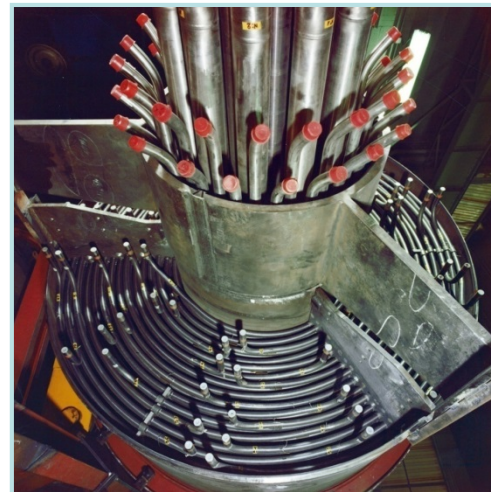
THTR-300 Steam Generator
