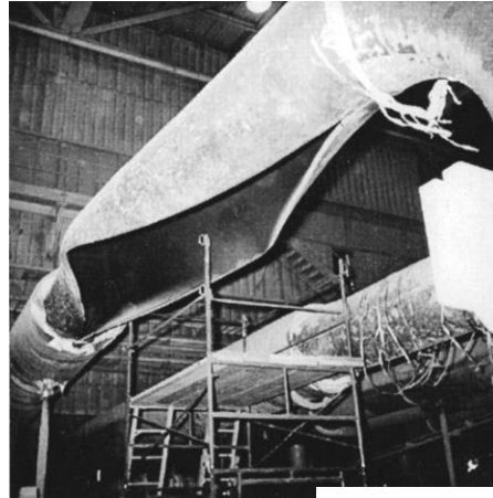
Seam pipe failure at coal power station (Viswanathan and Stringer, 2000)
