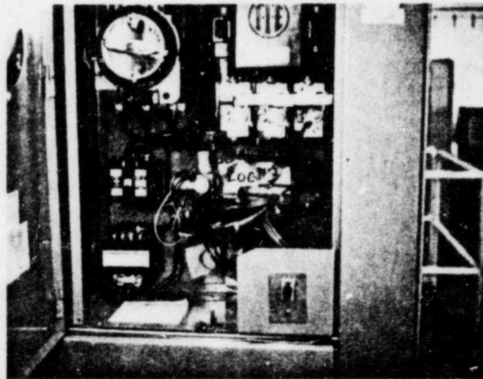
Figure IV.11 Accelerometer Location No. 2 During Full Level Testing
