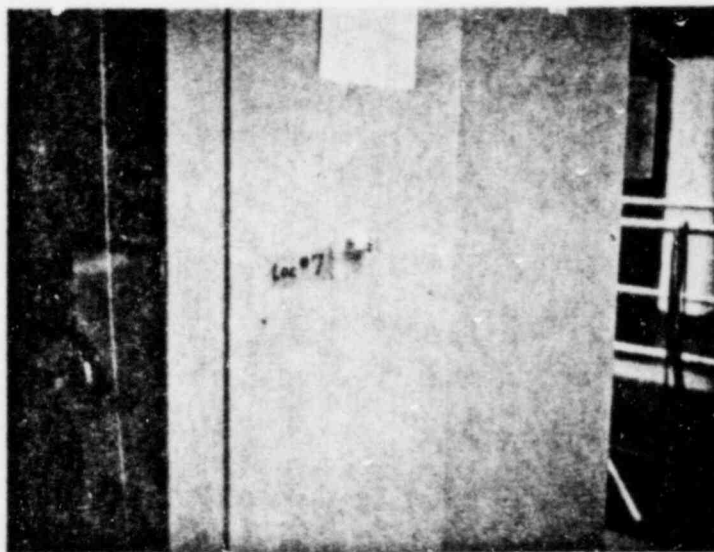
Figure IV.7 Accelerometer Location No. 7
