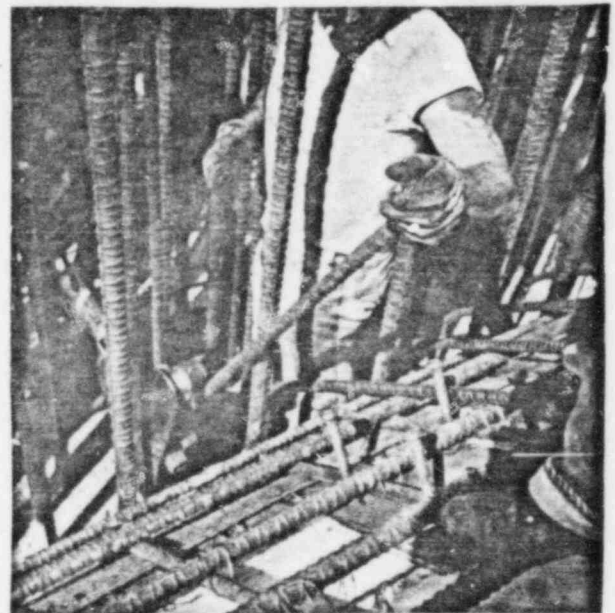
Figure 4 - Rebar being bent on the parapet of the shield building. Rebar is tied down before release of hydraulic pressure.
