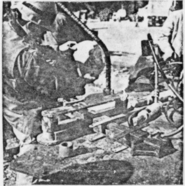
Figure 2 - Quality Control inspector uses template to examine bend radius. Bender frame in foreground.
