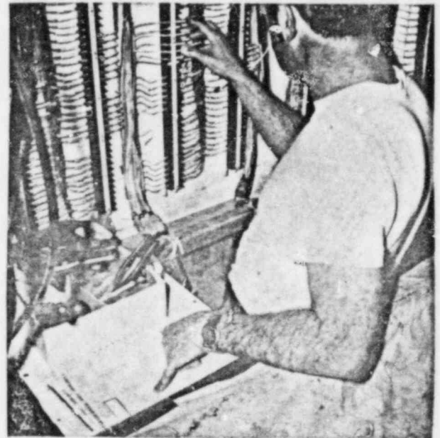
Figure 6 - Electrician terminating cables checks computer developed "termination card" against identified termination points.
