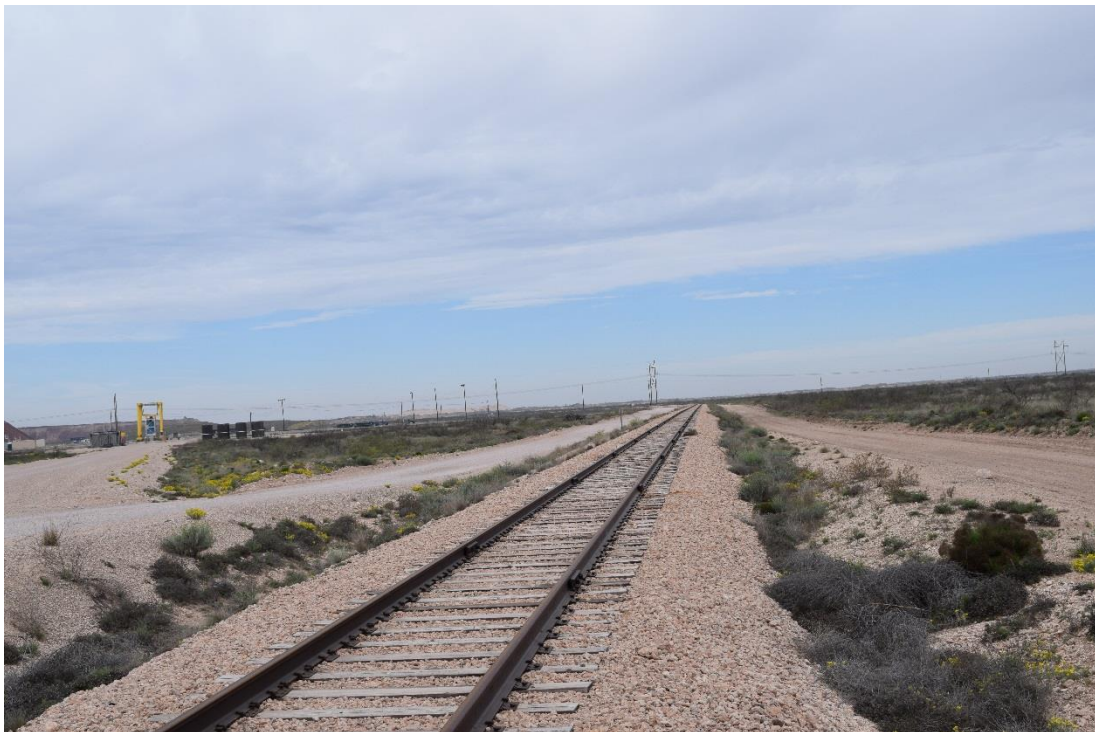
At P3, WCS railroad spur facing west towards New Mexico, south boundary of proposed site.
