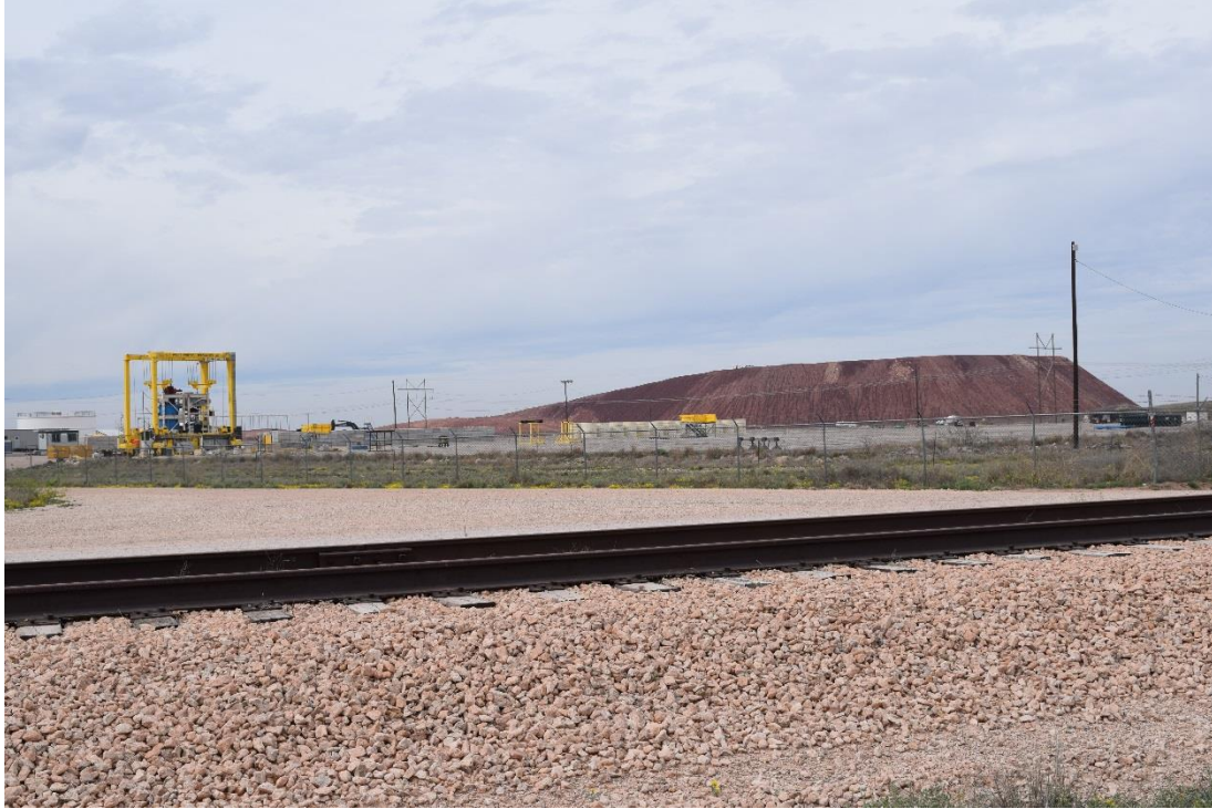
At P2, from south of new site facing southwest to redbed stockpile.
