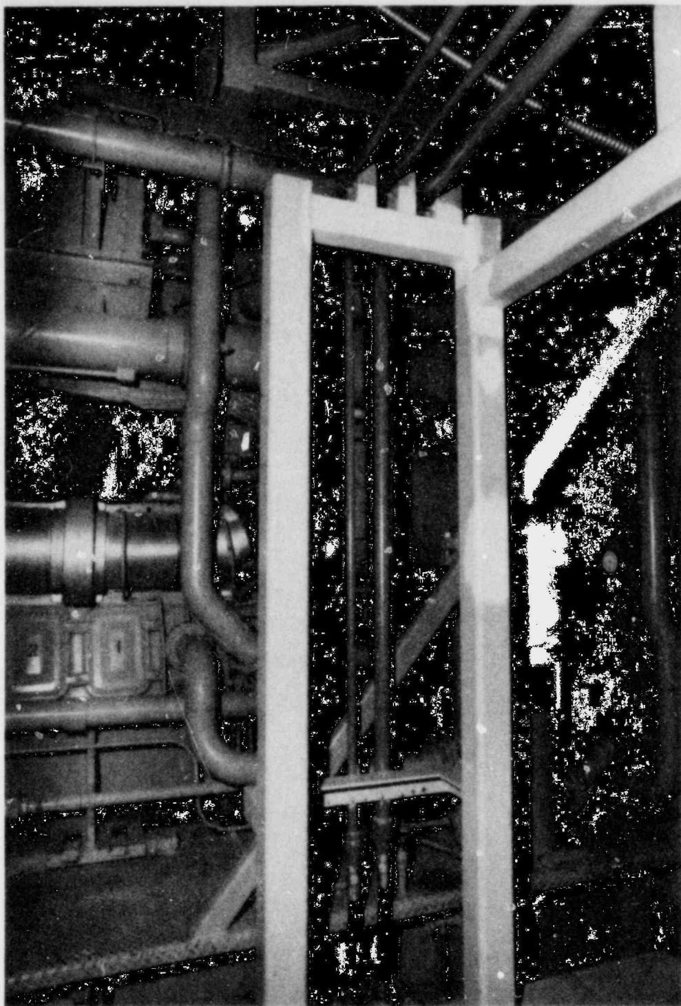
Figure 11. Diesel engine fuel lines (yellow) with seismic support.
