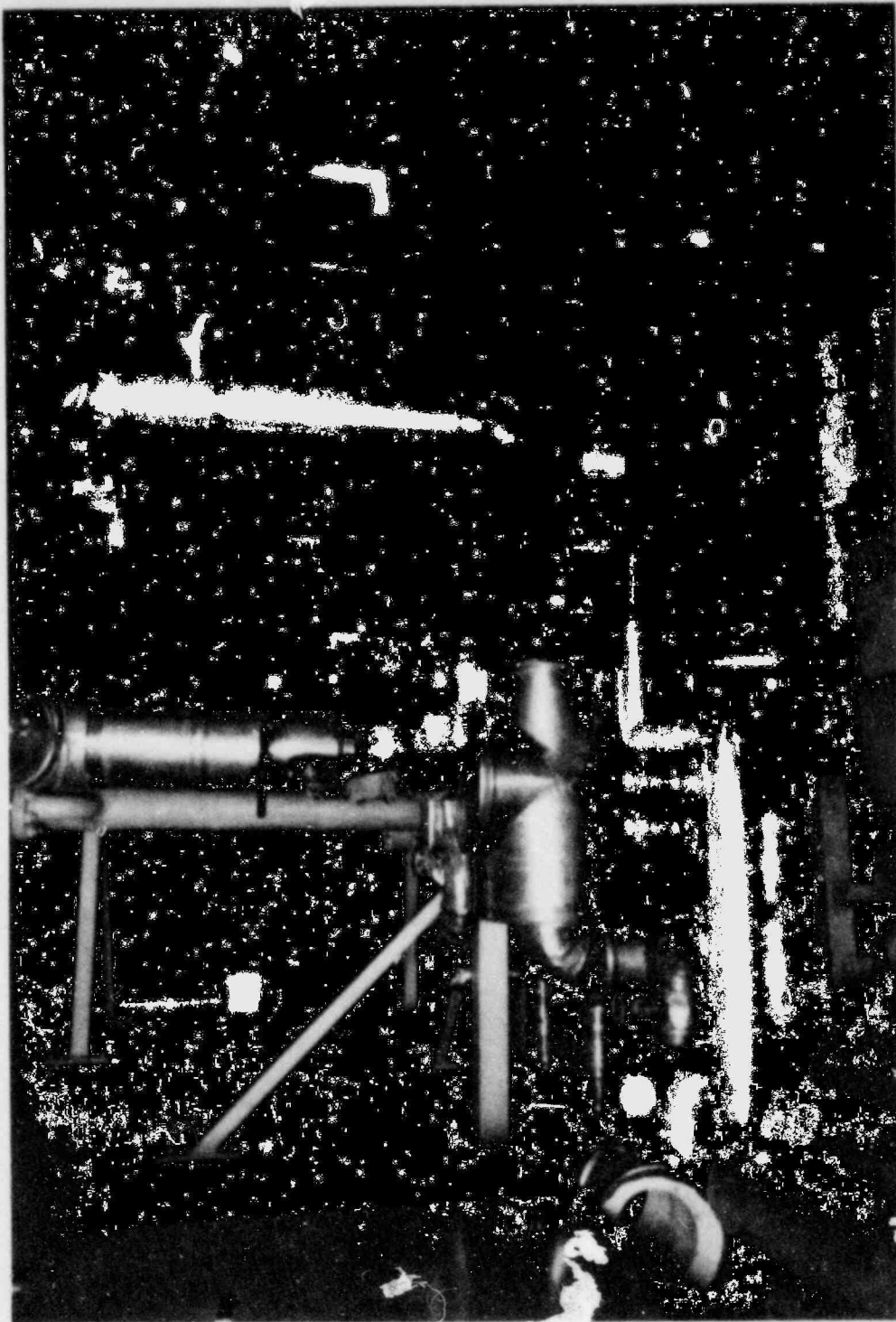
2. Turbine-driven auxiliary feedwater pump housed in a separate room.
