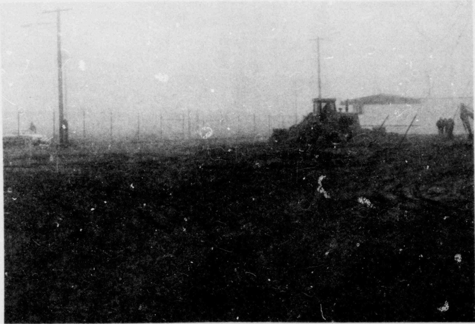
FIGURE 3. Excavation Progress for Steam Generator Examination Facility as of December 22, 1980
