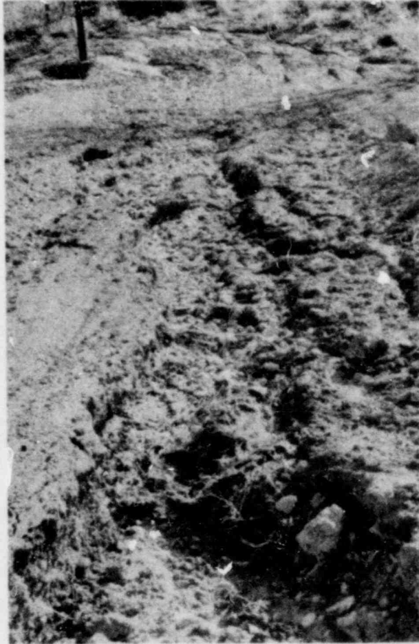
DRAINAGE AT SOUTH END OF SITE LOOKING SOUTH FROM T-11
