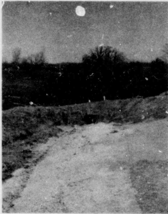
DRAINAGE CULVERT LOOKING NORTH
