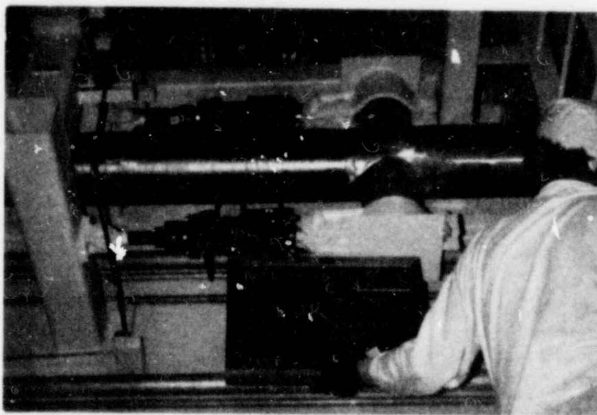
Figure A.19 Hydraulic snubber, piston fully extended
