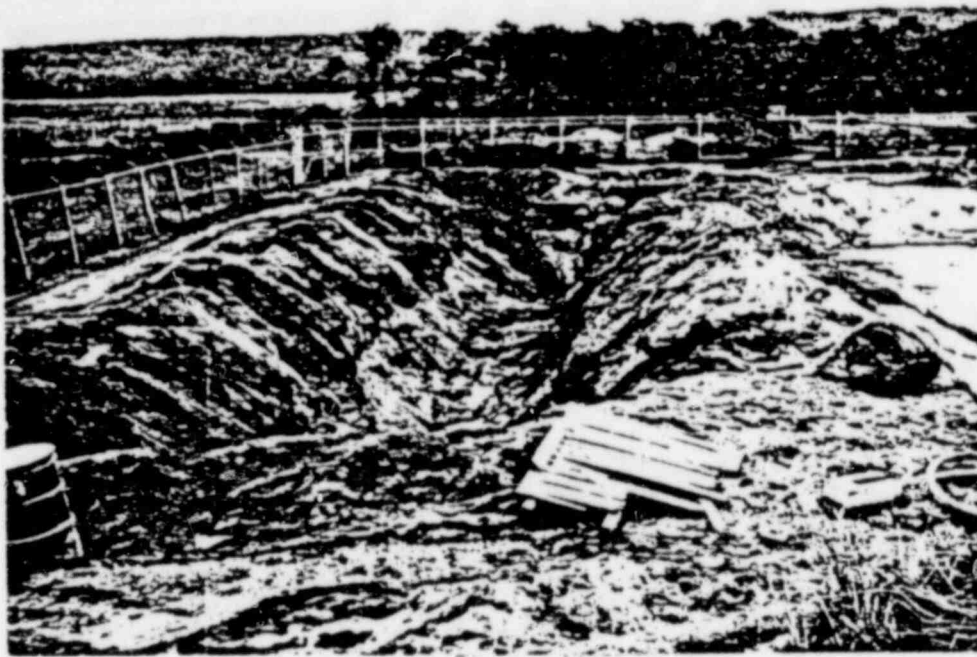
Photograph 5 - Hole left after removal of lagoon C
