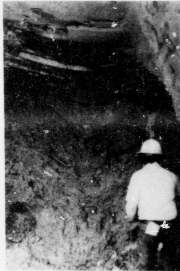
b. Weathering of infilling material
