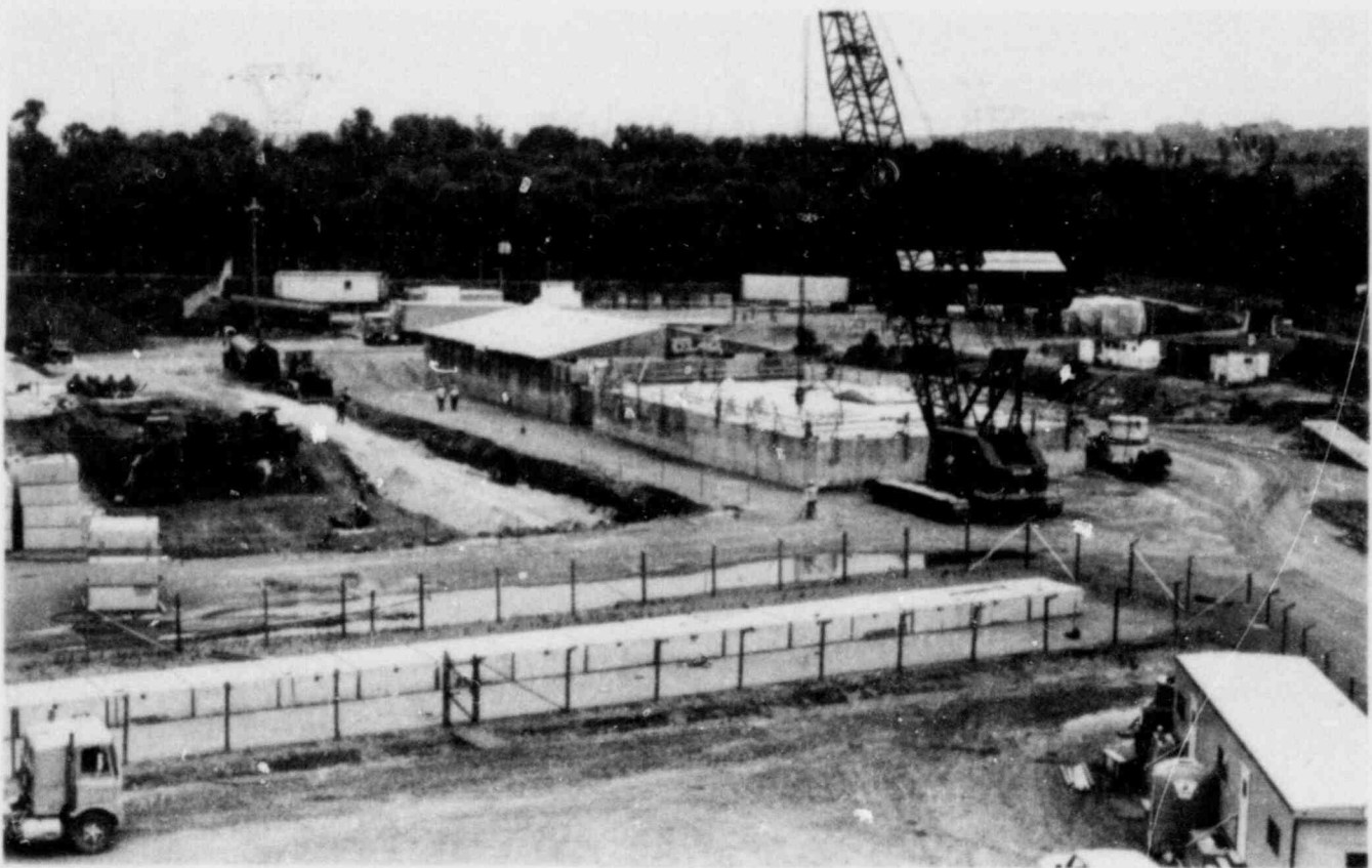
Storage area at Three Mile Island for "spent" ion-exchange resin liners containing radioactive material removed from the contaminated water in the auxiliary building tanks at the TMI-2 site. One modular storage structure is shown at left center of photo, while construction of a new facility next to it is under-
