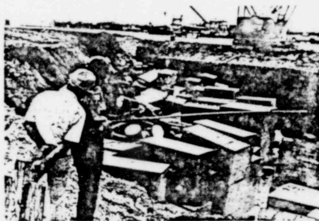
This "fish pole" radiation survey meter permits inspectors to accurately assess the radioactivity of low-level waste material in trenches prior to burial. Containers have just been delivered and dumped by trucks in background and will be covered by earth-moving equipment as soon as radiation levels and distribution have been recorded.
