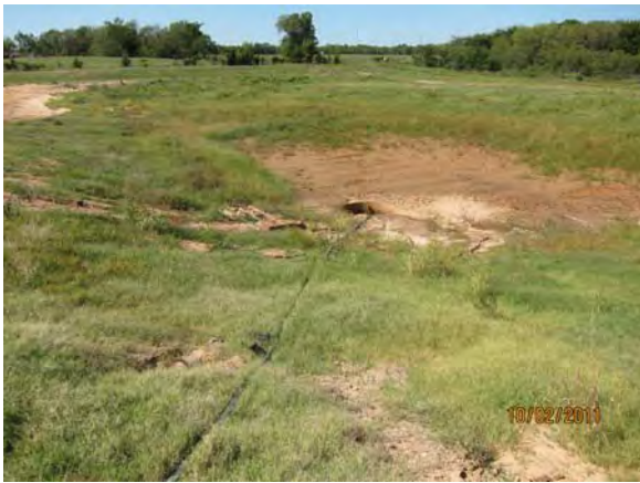
Figure 1 - Pond 3, looking to the north west
