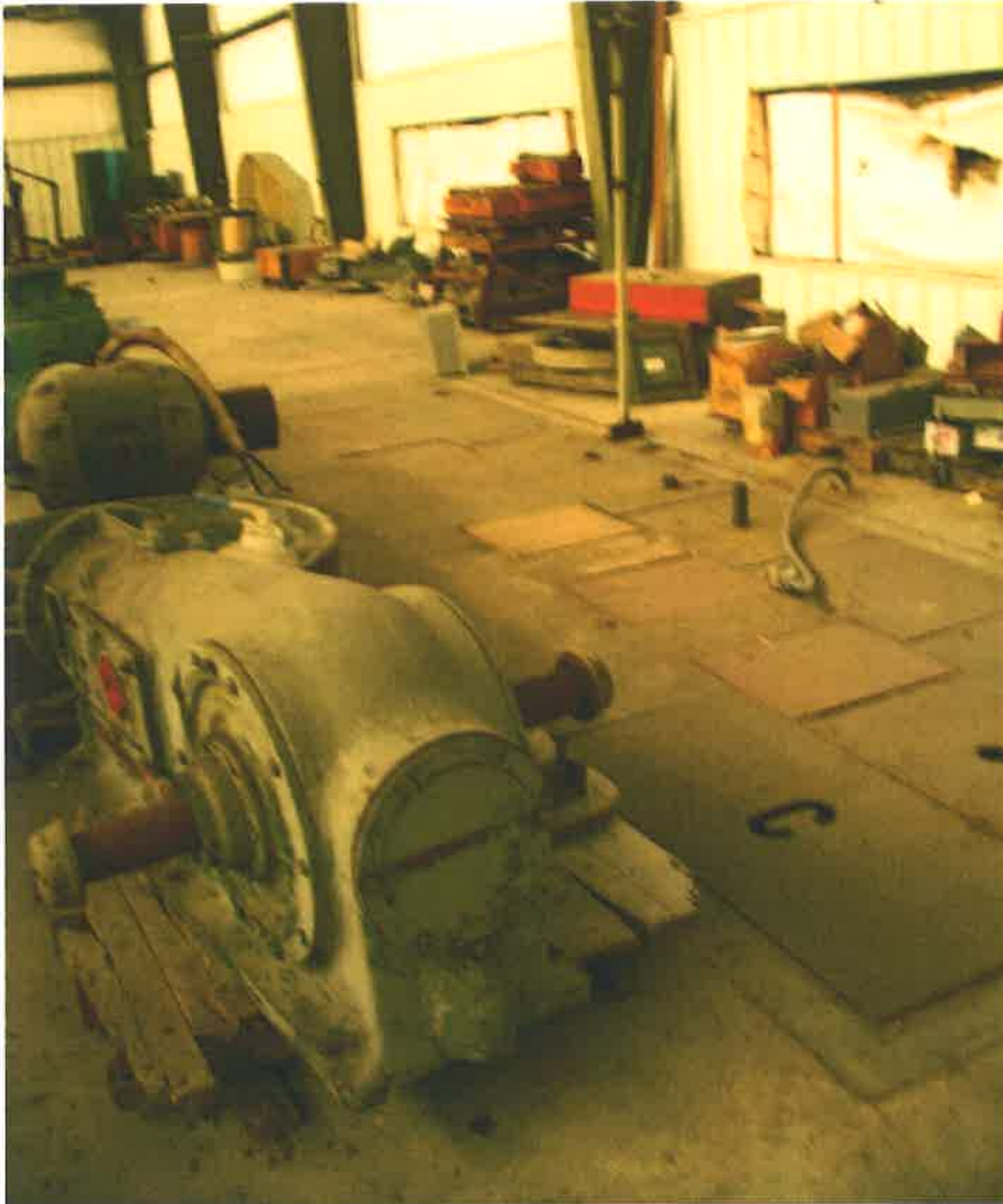
Inside west side of Electron Beam Building, showing stored equipment and furniture, and steel plates covering cooling water reservoir. (9/27/2005)
