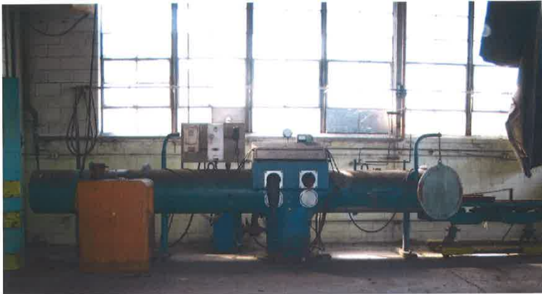
Vacuum Box for working with sintered shapes, west end Sintering Building (9/27/2005, subsequently removed)
