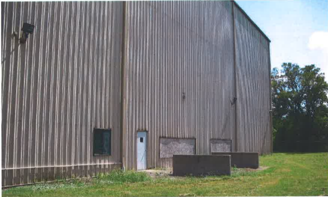
West end, Electron Beam Building (9/27/2005)
