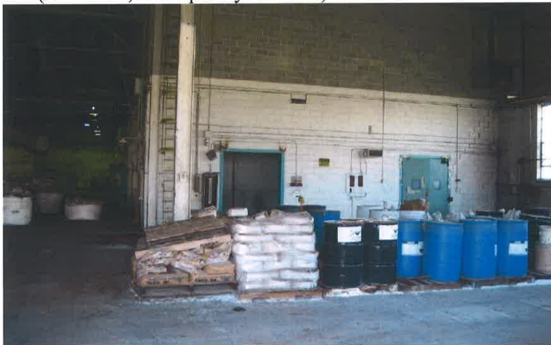
Drums and sacks of chemicals stored inside Sintering Building, east end looking west (9/27/2005, subsequently removed)
