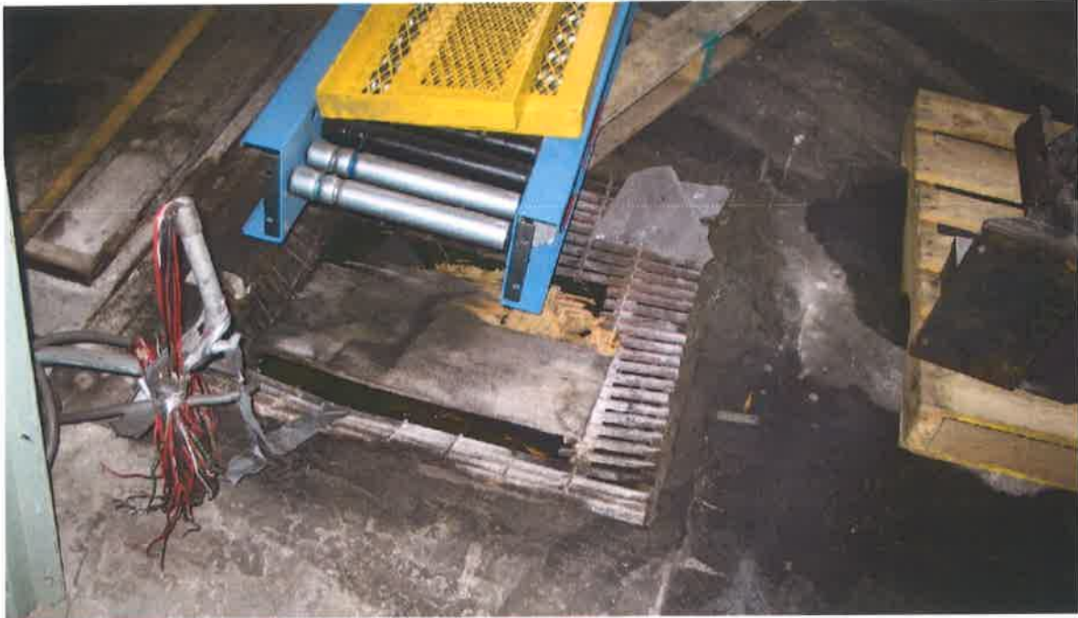
Pallet of newly-fabricated steel parts and conveyor near floor drain near east end of Sintering Building (10/27/2006)
