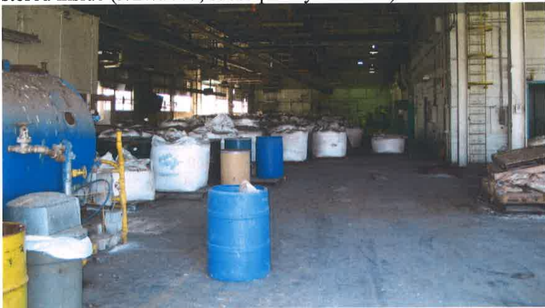
Sintering Building, south end, showing drums and super sacks of chemicals stored inside (9/27/2005, subsequently removed)
