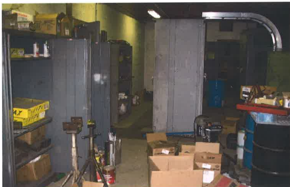
Equipment/materials storage room in Electron Beam Building. Note electrical equipment (transformer?) in background (10/27/2006)
