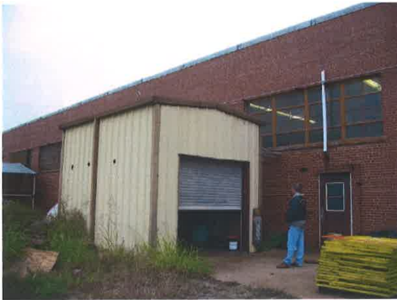
Building 6, South of Service Building, from southeast (10/27/2006)
