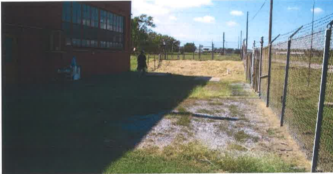
North side of Sintering Building, looking west, showing above-ground line leading off to west.
