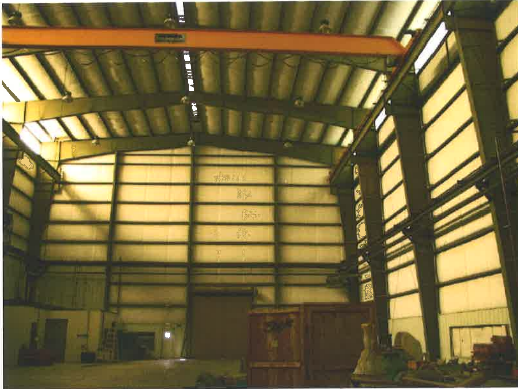
Interior of Electron Beam Building, looking south, showing overhead crane. (9/27/2005)
