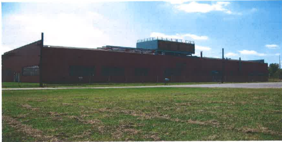
Sintering Building from the Northwest, showing cooling tower on roof
