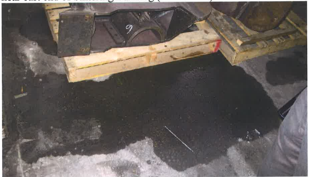
Oil stained concrete near pallet of newly-fabricated steel parts
