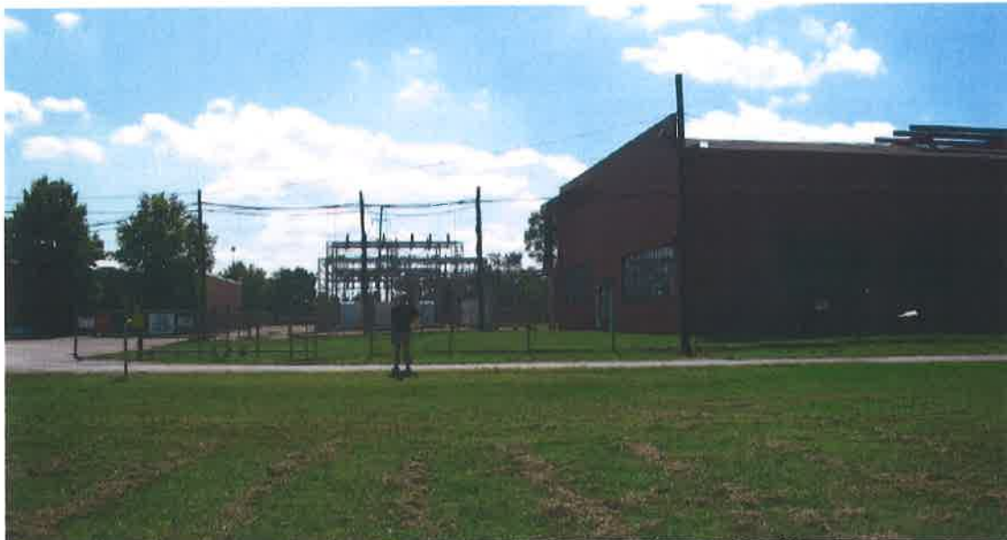
Electrical Substation & Sintering Building, from North
