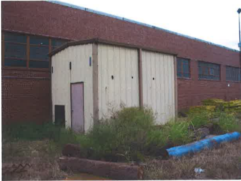
Building 6, South of Service Building, from southwest (10/27/2006)
