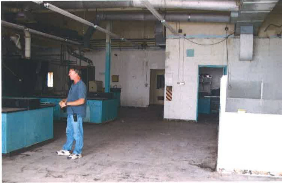
Laboratory in Service Building Looking North (9/27/2005)
