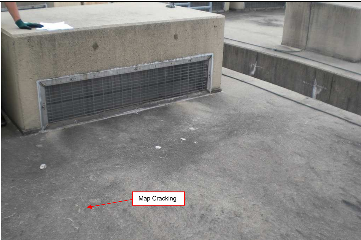
Photograph 8. Top of HSM 31 showing map cracking.
