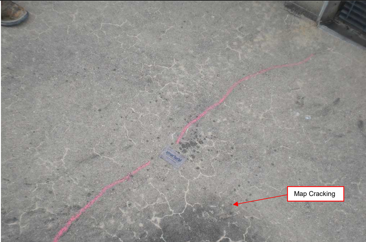
Photograph 9. Top of HSM 46 showing map cracking and shrinkage cracking.
