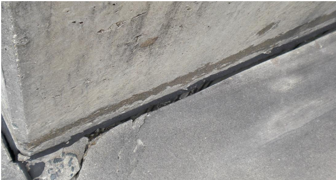
Figure 26 – Failed Seal Material at Grade Slabs
