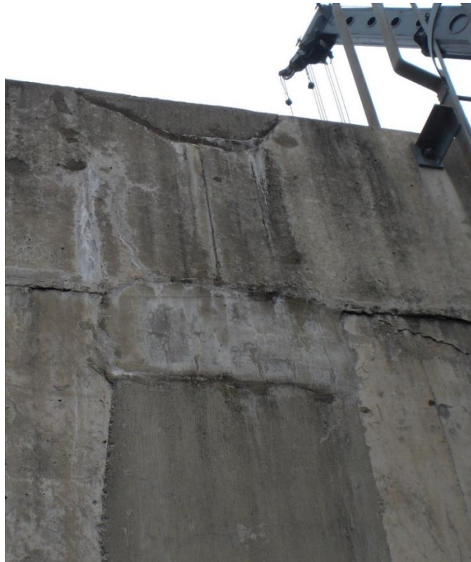
Figure 15 – Efflorescence Observed in Previous Repair Areas on the Side of HSM-1
