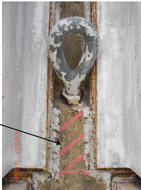
Figure 22 – Possible Delamination Below Cask Restraint Assembly Turnbuckle Eyes
