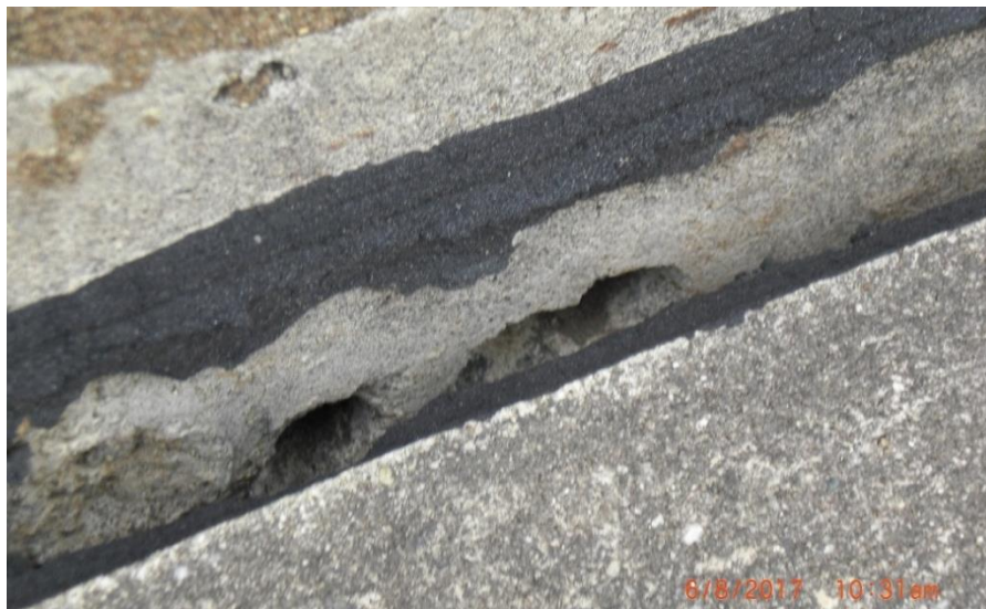
Figure 25 – Indentation in HSM-37 Near Failed Grade Slab Seal
