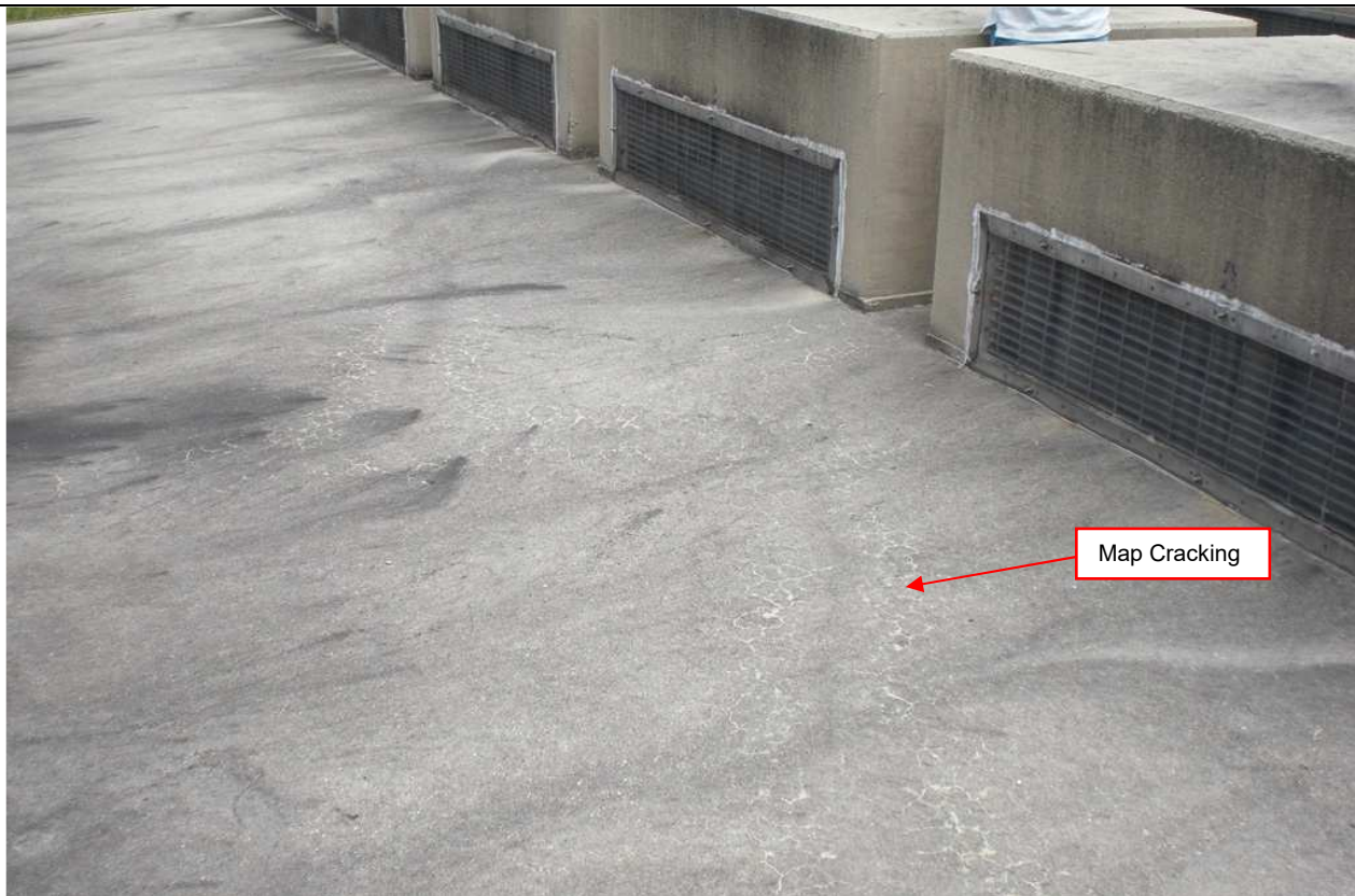
Photograph 6. Top of HSM 7 showing map cracking.
