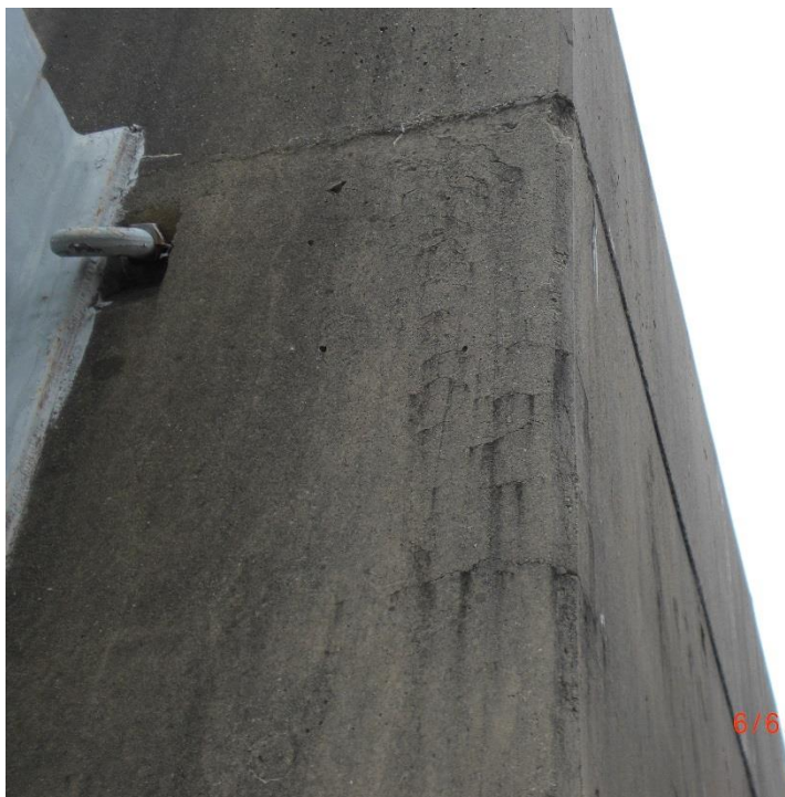
Figure 12 – Map Cracking on the Wall Corner of HSM-7
