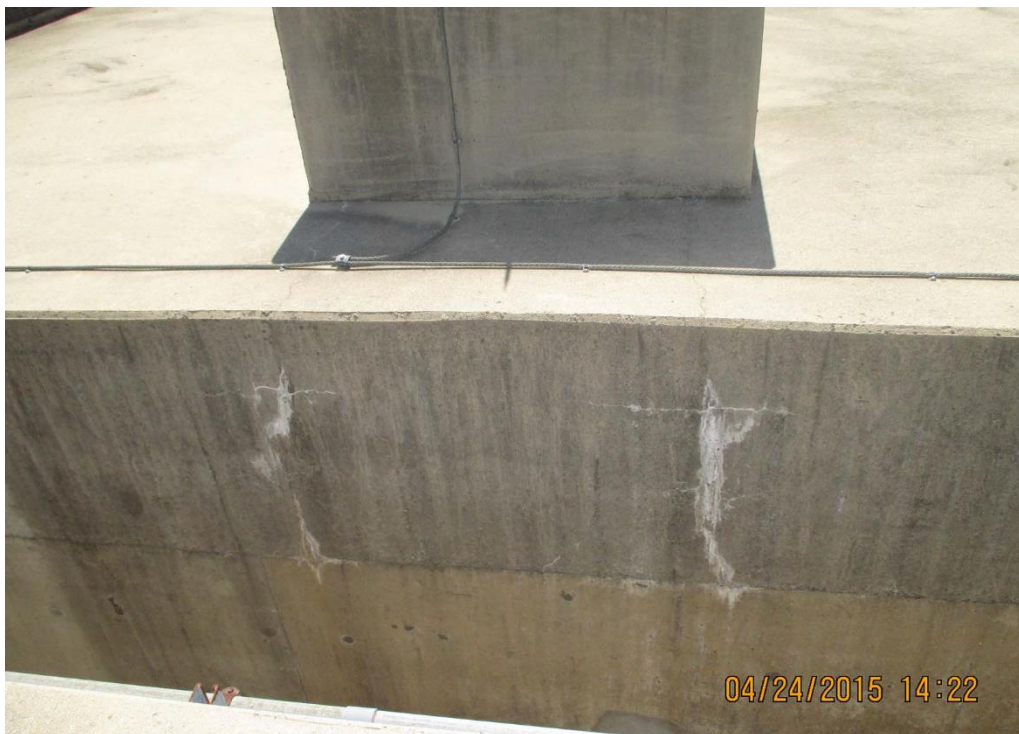
Figure 10 – Prior 2015 Site Annual Inspection Showing Similar Cracking and Efflorescence as in Figure 9
