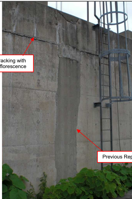
Photograph 4. West face of HSM 1 and 13 showing previous repairs and cracking with efflorescence.
