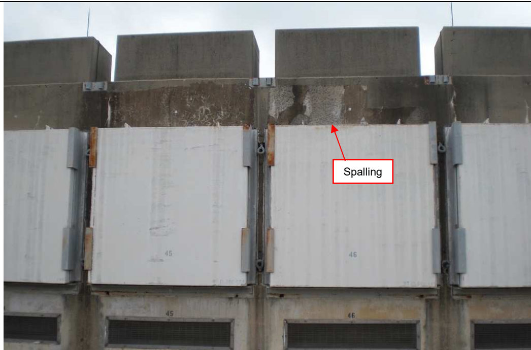
Photograph 2. HSMs 45 and 46 showing failed repairs and spalling.
