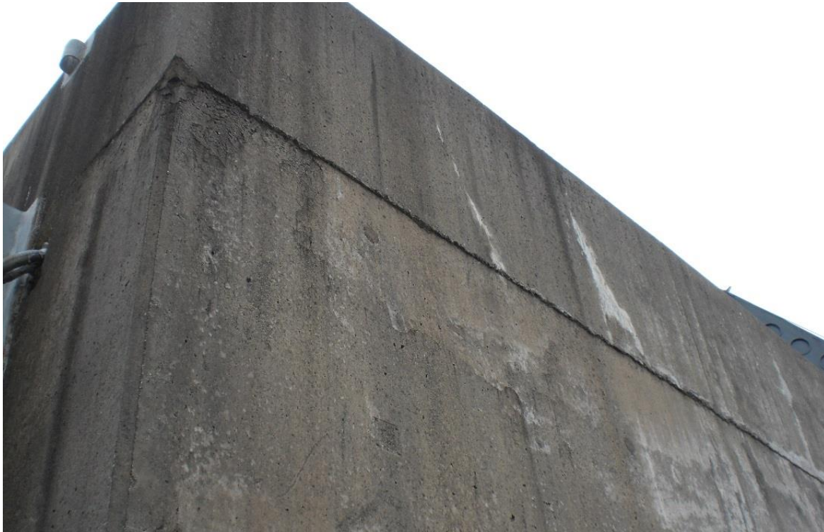
Figure 13 – Map Cracking on Wall of HSM-1
