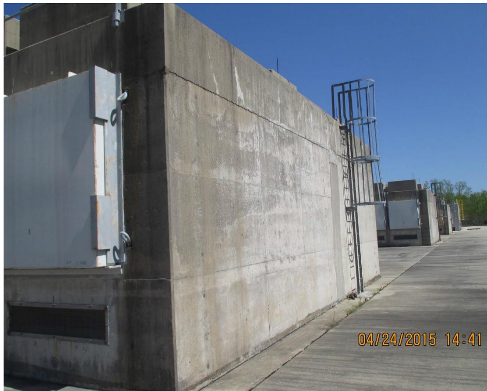
Figure 14 – Prior 2015 Site Annual Inspection Showing Prior Condition of HSM-1 Walls
