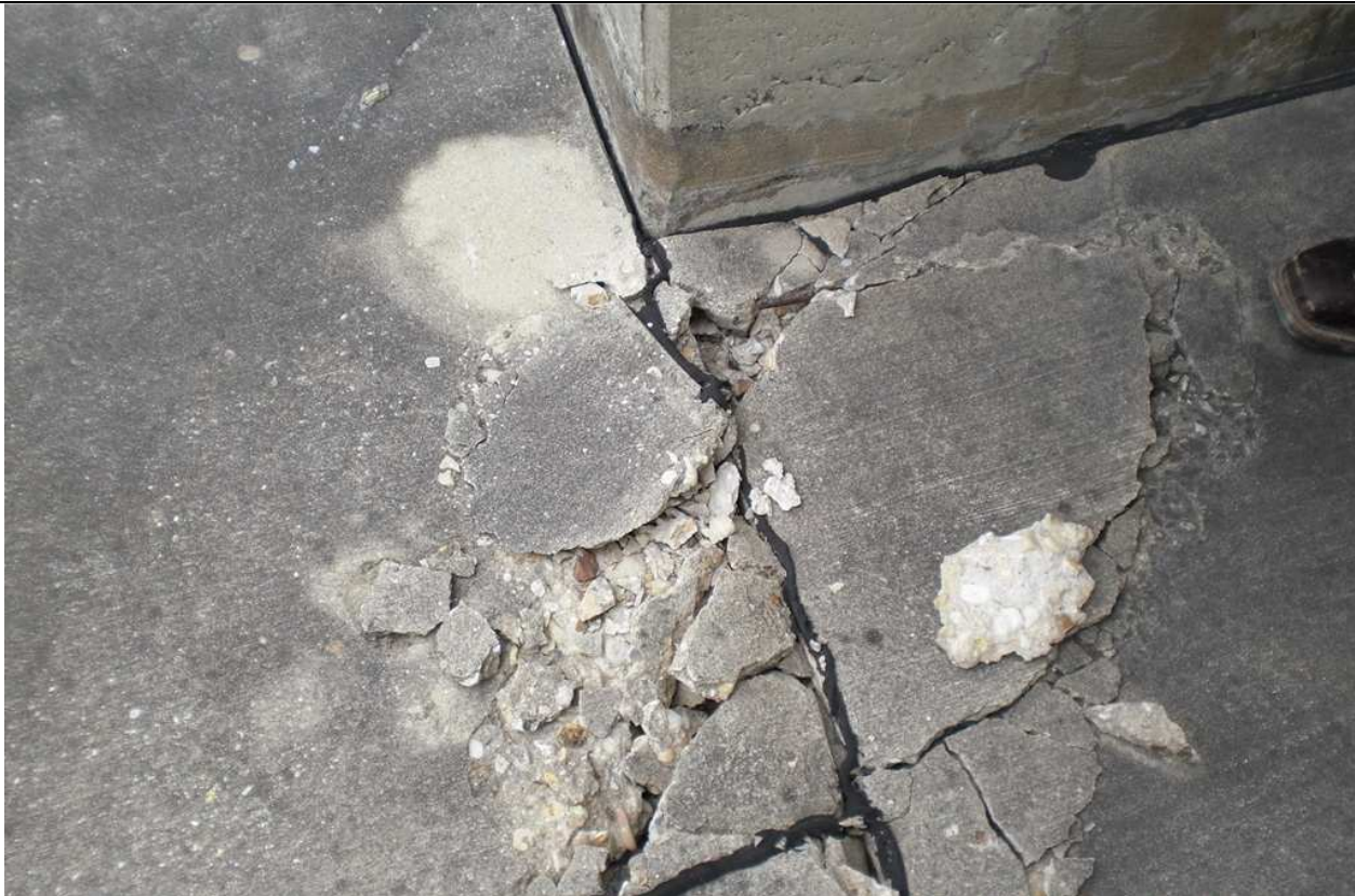
Photograph 10. Ground slab on the northwest corner of HSM 31 showing delaminated and spalled concrete.
