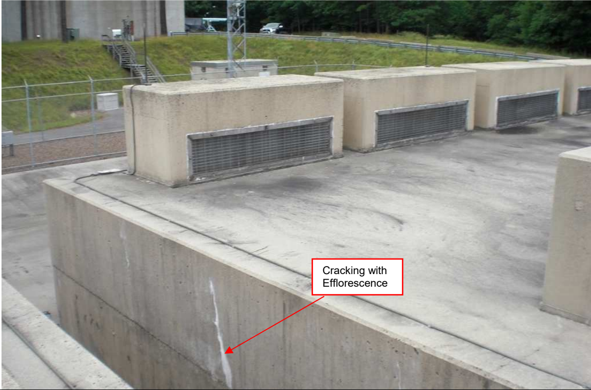
Photograph 7. West face and top of HSM 7 showing cracking with efflorescence.
