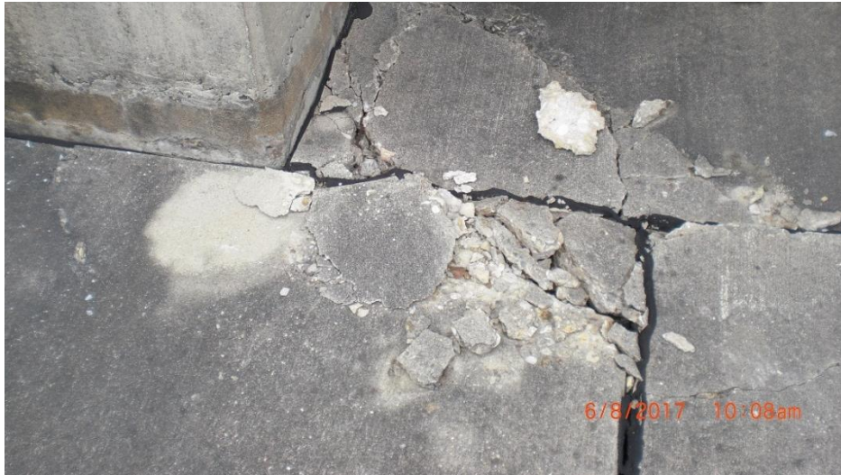
Figure 24 – Grade Slab Damage
