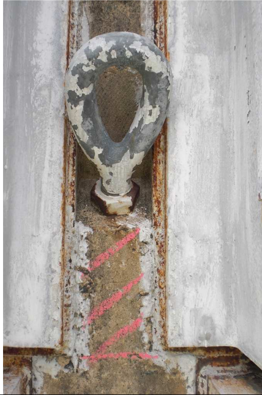
Photograph 11. South face of HSM 46 showing delaminated concrete.
