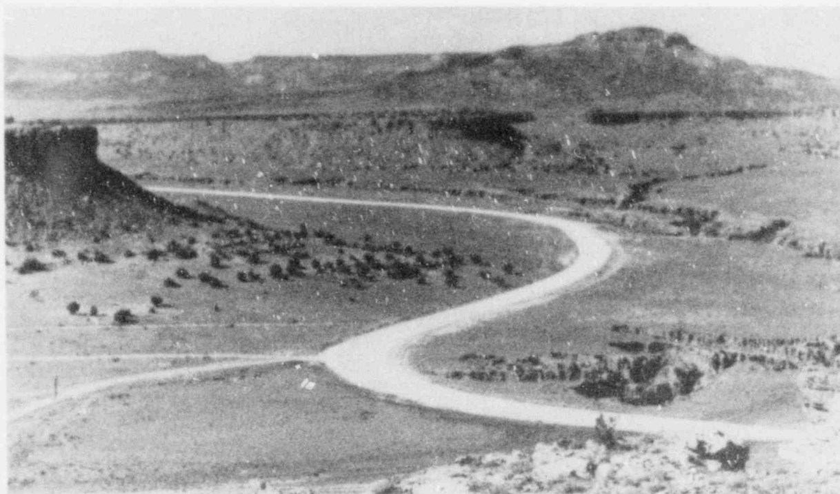
Figure 2. View of the St. Anthony Erosion Plane.
