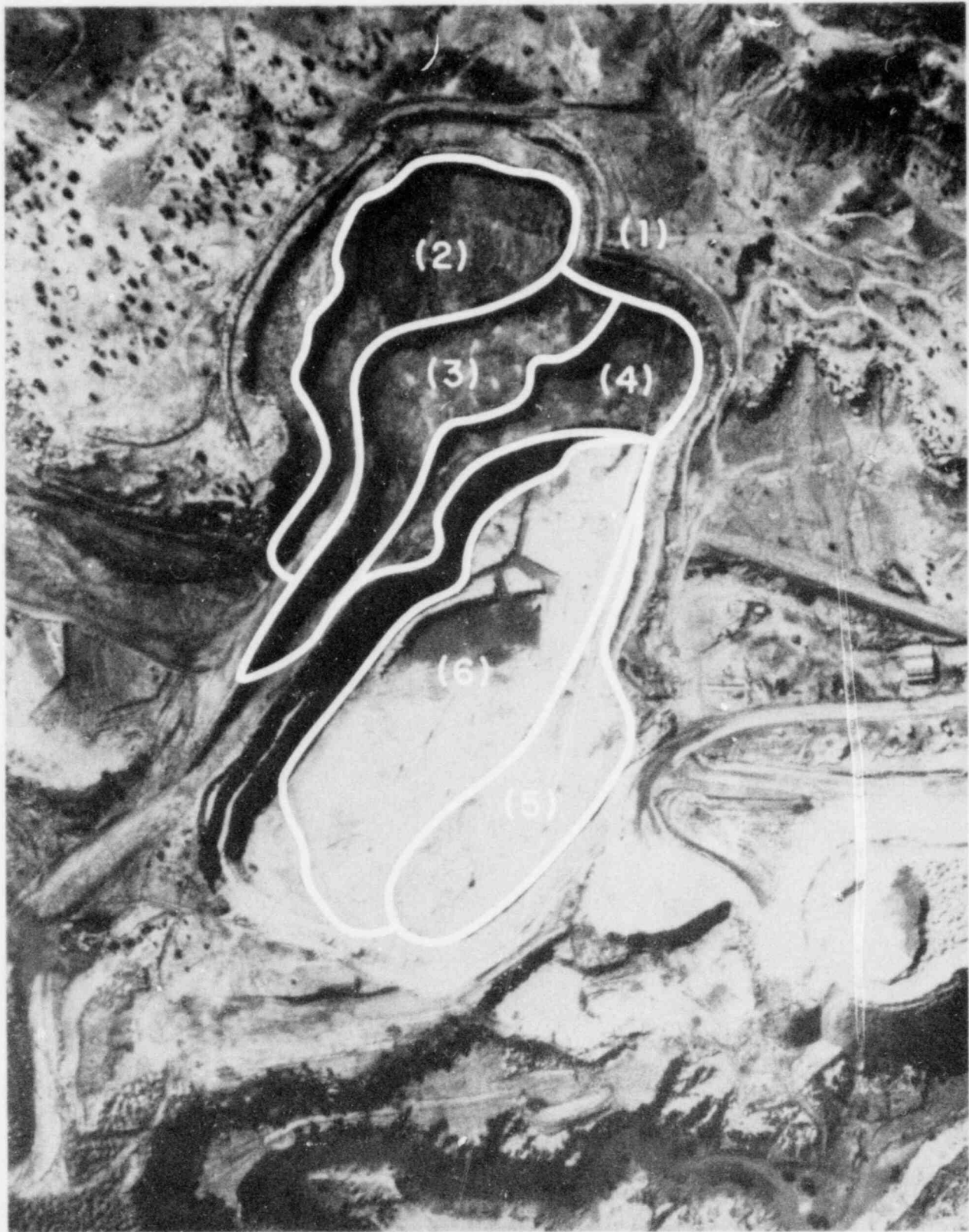
Figure 21. Enlarged Aerial View of the Inactive Pit Showing the Different Levels.
