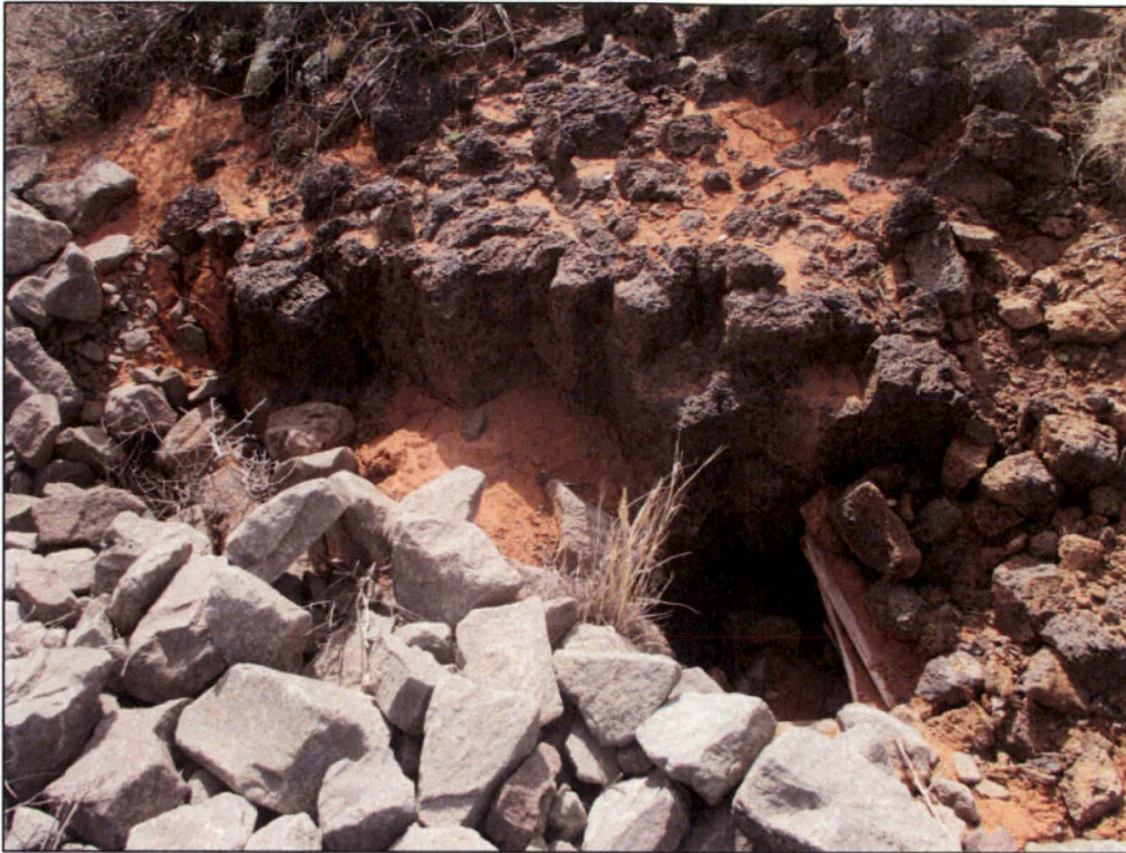
PL-17. Settlement in Fill Covering Basalt at the Interface of the East Dump Cover
