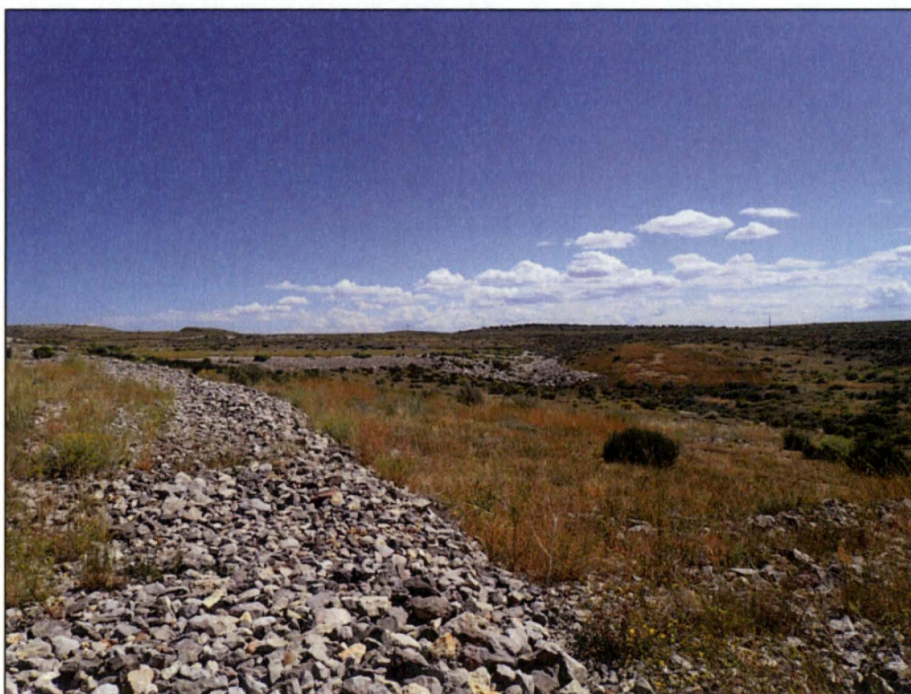
PL-18. Erosion Protection Rock Berm with Ancillary Cell and Diversion Channel No. 2 in Background
