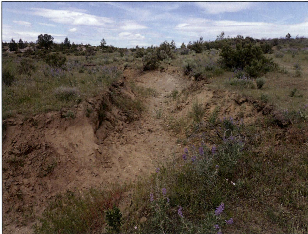
PL-6. Gully Downgradient of Riprap-Armored Swale (Near Perimeter Sign P1)
