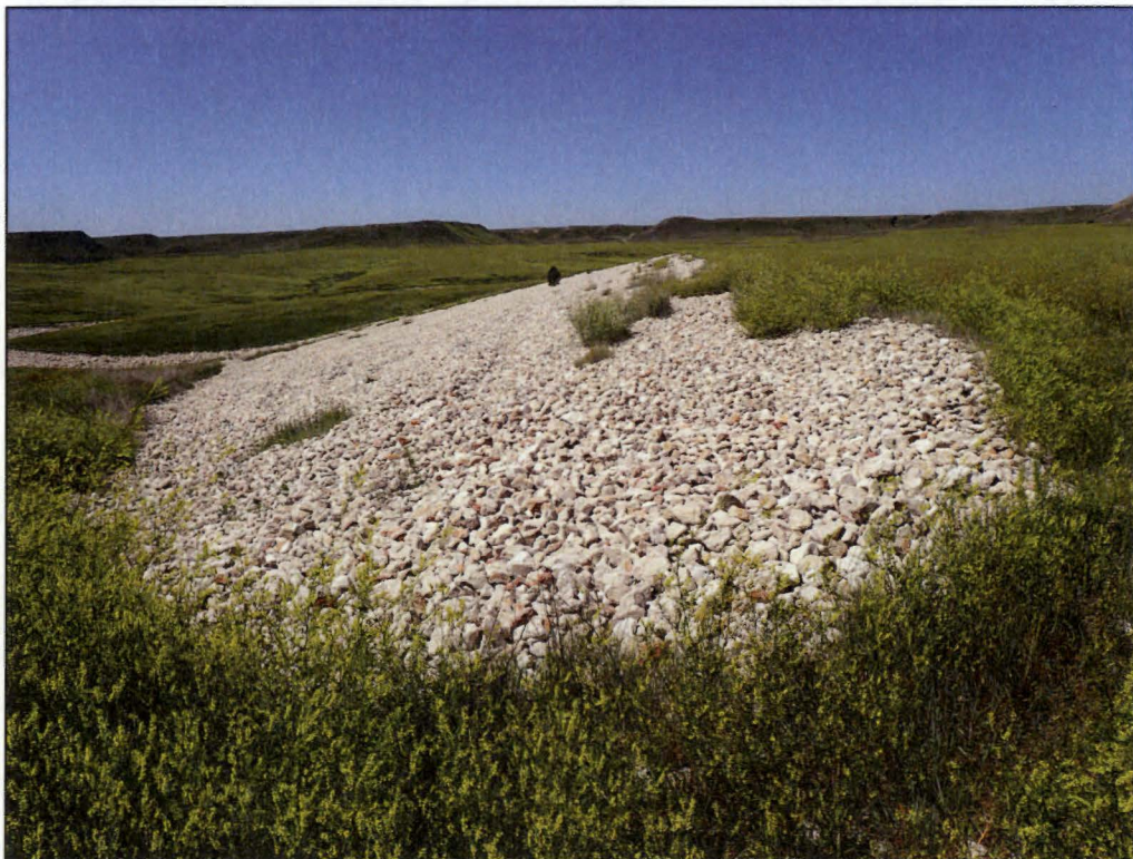
PL-8. East Portion of Containment Dam
