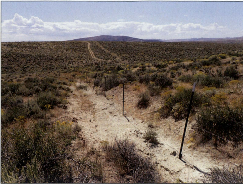
PL-1. Erosion Along Southwest Perimeter Fence
