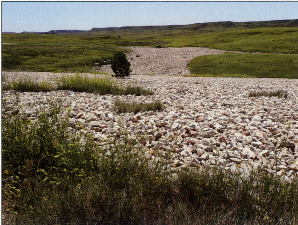
PL-7. Center of Containment Dam and Drainage Channel
