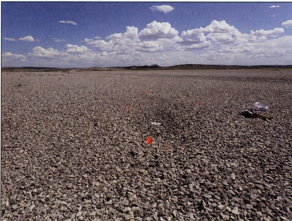
PL-6. Depression Feature on Top of Disposal Cell
