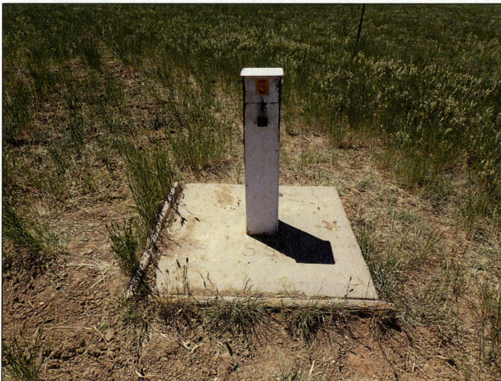
PL-6. Monitoring Well 5-SC
