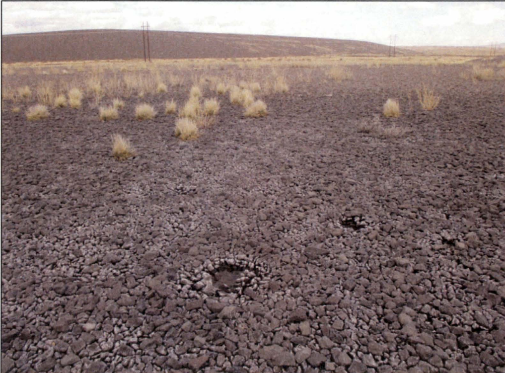
PL-12. Minor Ponding in the Shallow Depression on the Northwest Extension of the Carbonate Tailings Disposal Cell
