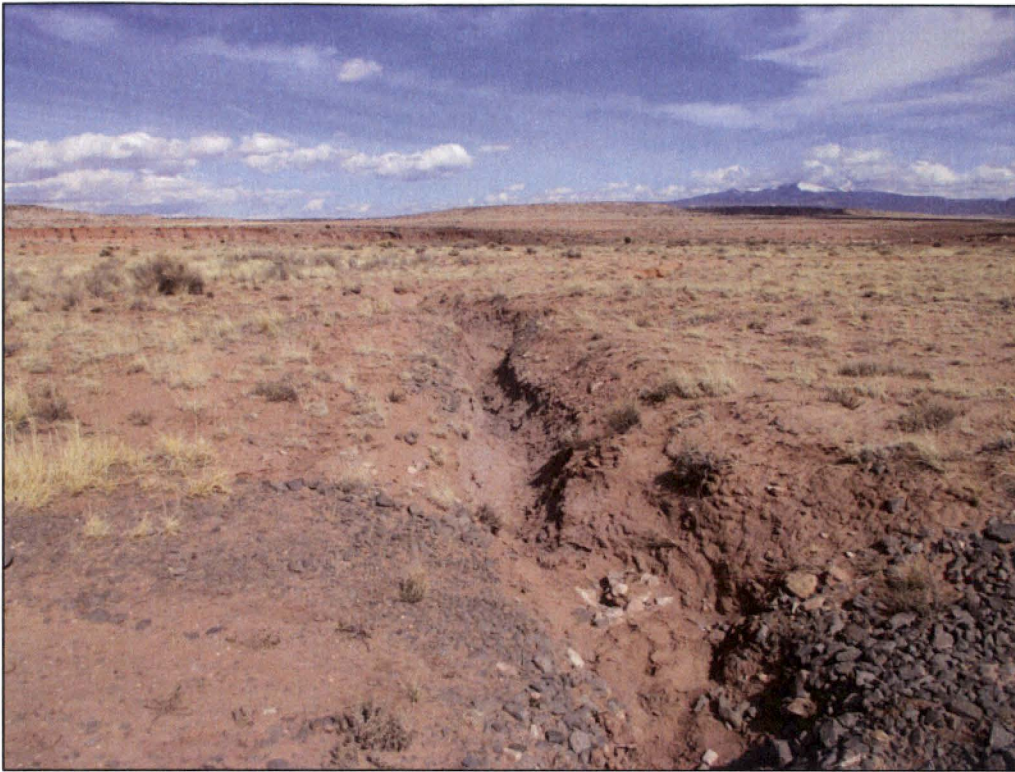
PL-1. Erosion of the Site Perimeter Road (South Area)
