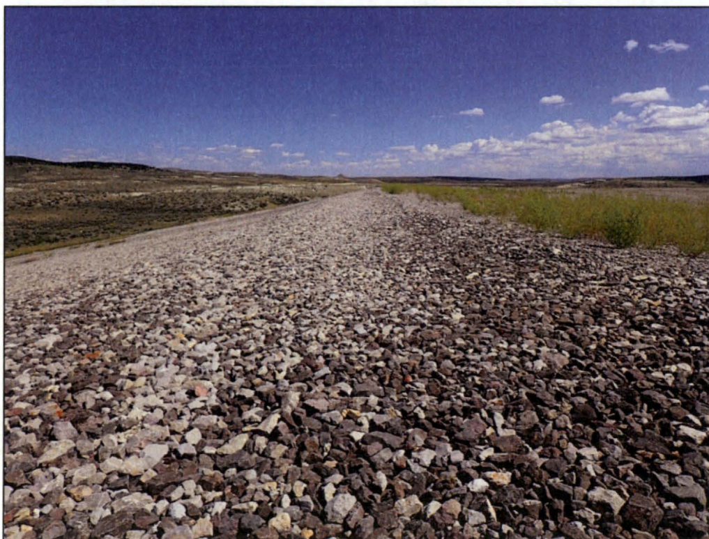
PL-10. Intersection of Disposal Cell Top Slope and North Side Slope
