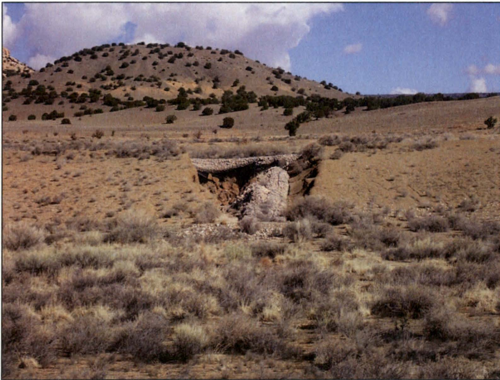
PL-14. Runoff Control Structure G
