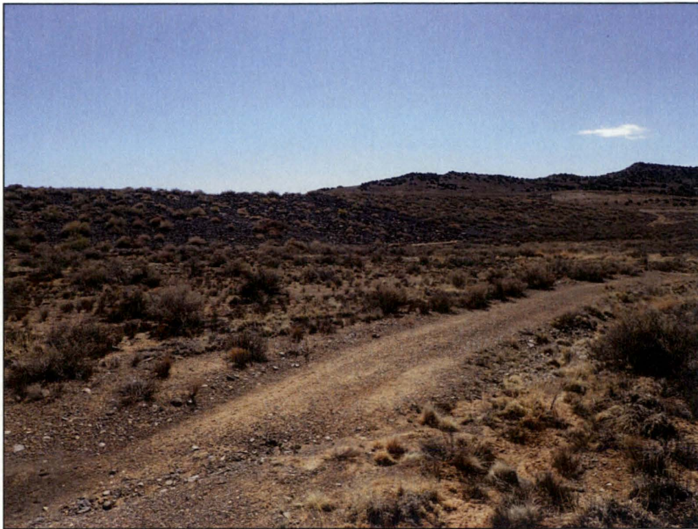
PL-9. Containment Dam Spillway
