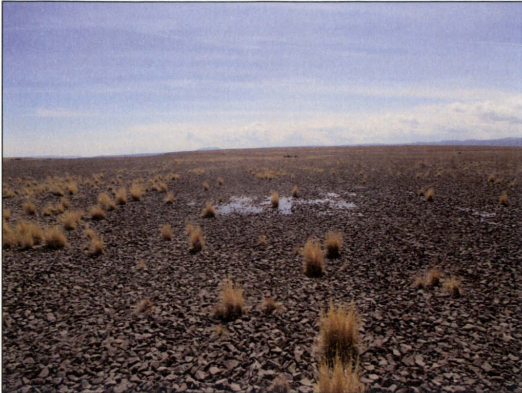
PL-7. Ponding on the Top Slope of the Main Tailings Disposal Cell
