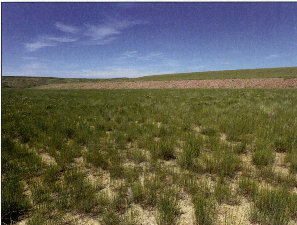
PL-10. Disposal Cell Dam Outslope
