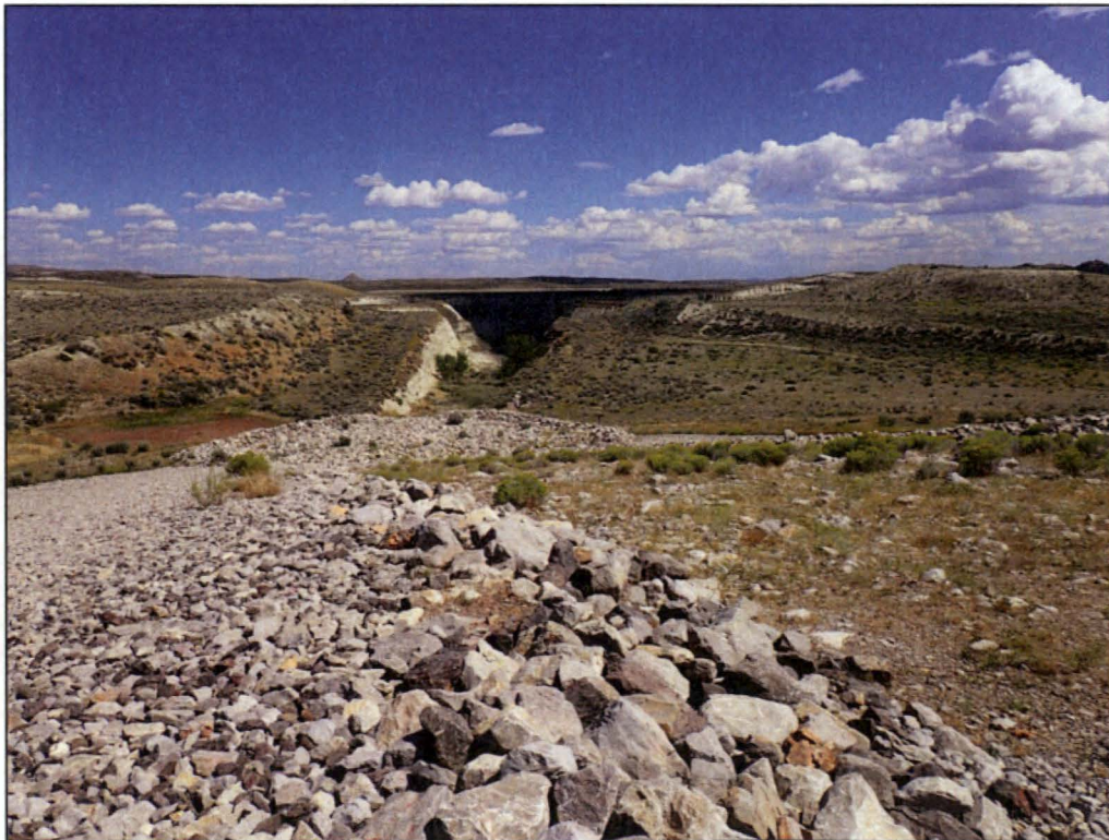
PL-16. Launch Rock Erosion Protection Basin on Disposal Cell East Side Slope; Rob Pit in Background
