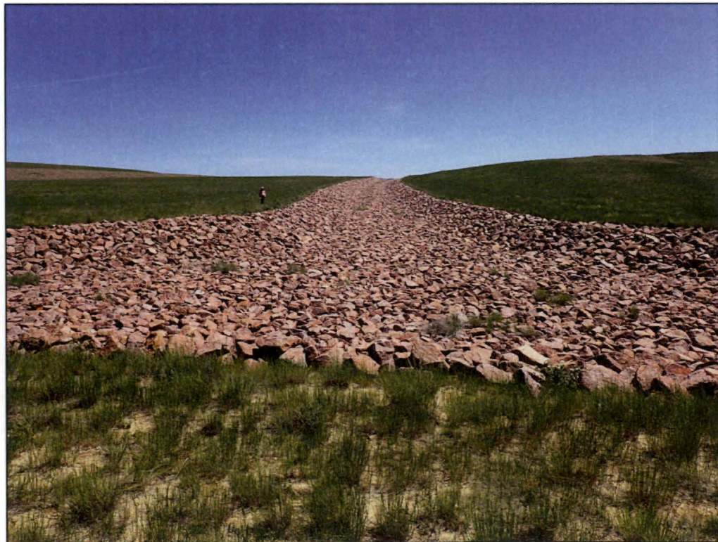
PL-12. Riprap-Armored Diversion Channel
