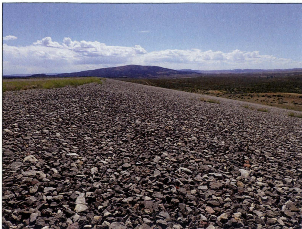
PL-9. Intersection of Disposal Cell Top Slope and West Side Slope
