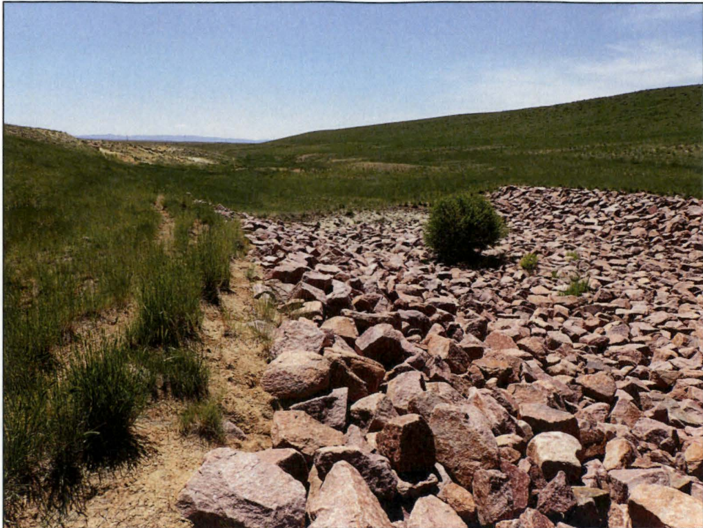
PL-13. Outlet of Riprap-Armored Diversion Channel
