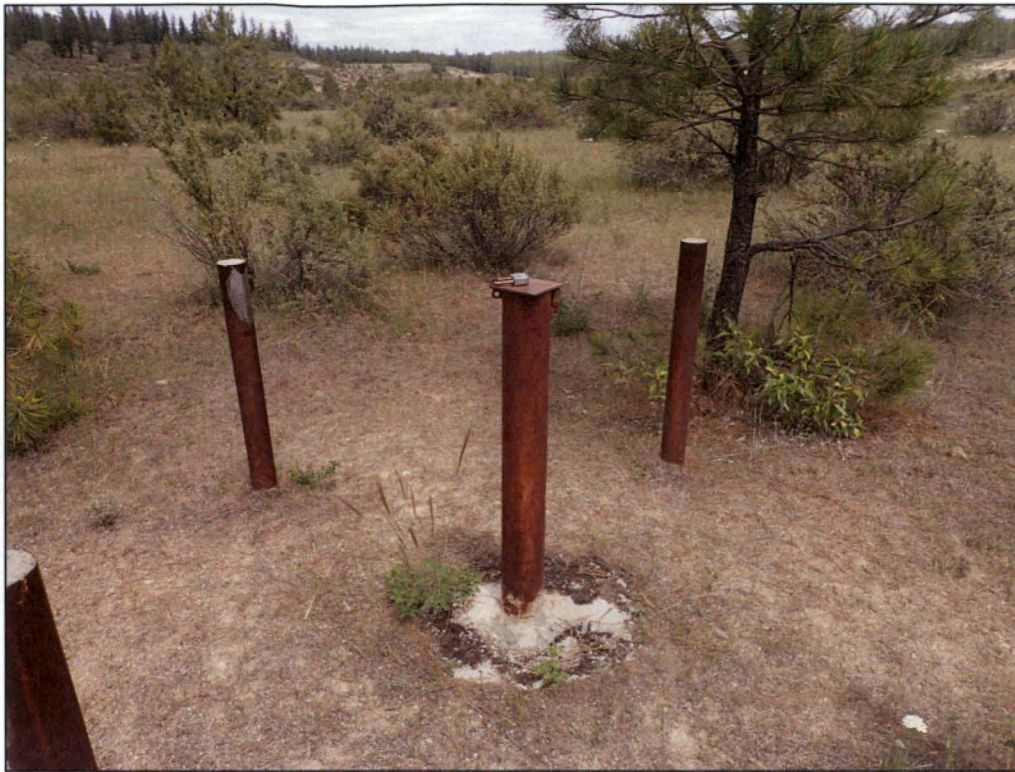
PL-5. Piezometer PZ-1
