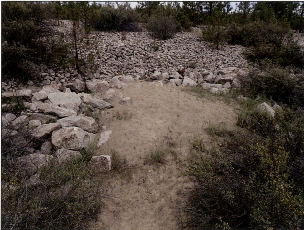
PL-8. Sand Deposit at Toe of Containment Dam Outslope
