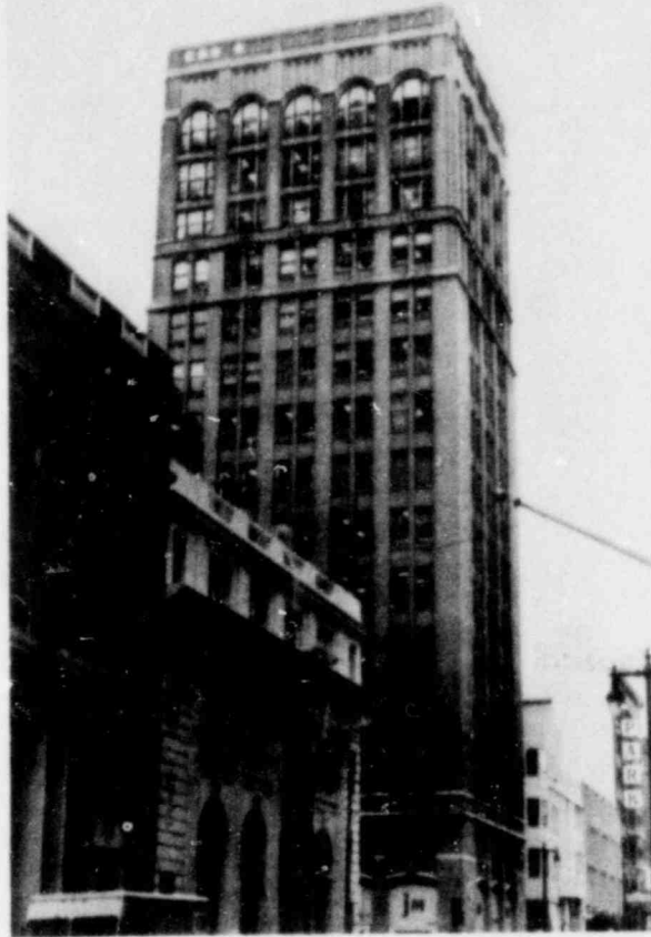
155 Montgomery St., East Elevation from Bush Street
