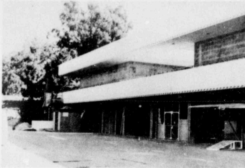
Arts Building 534, Basement and First Floor View to Northeast
